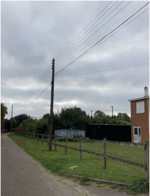
Figure. 25 | Existing telegraph posts.
