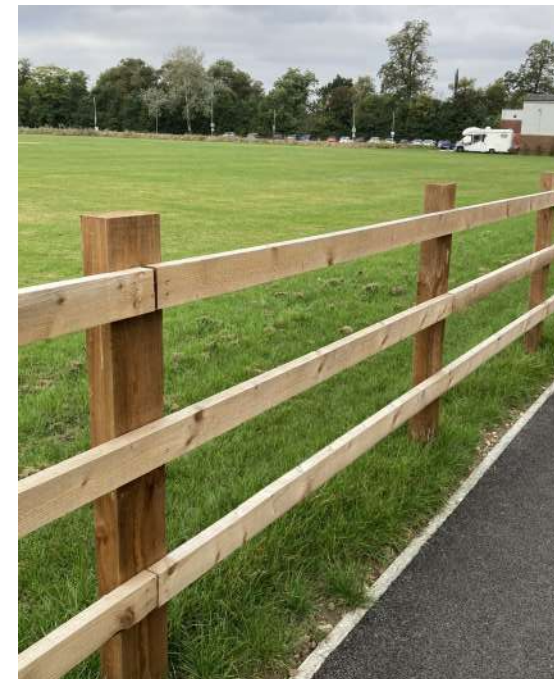
Figure. 21 | Existing post and rail fencing to be extended.
