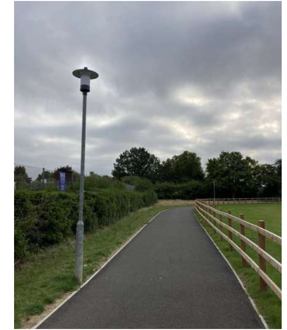
Figure. 18 | Existing asphalt pedestrian path to 3G Pitches.
