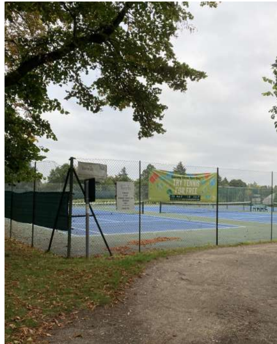
Figure. 10 | Existing Sonning Lawn Tennis Club courts.
