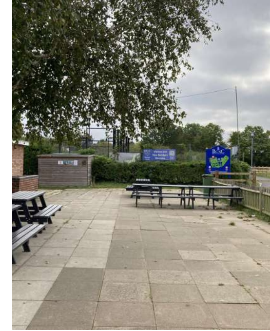
Figure. 22 | Existing pedestrian approach to courts via social space.
