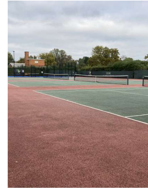
Figure. 32 | Existing hardstanding for existing tennis courts.
