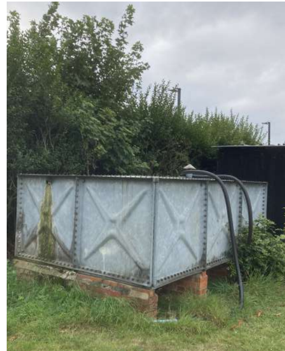
Figure. 11 | Existing tank to be removed adjacent to existing padel courts.
