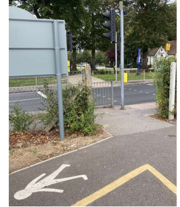
Figure. 23 | Existing safe pedestrian access point off Sonning Lane.
