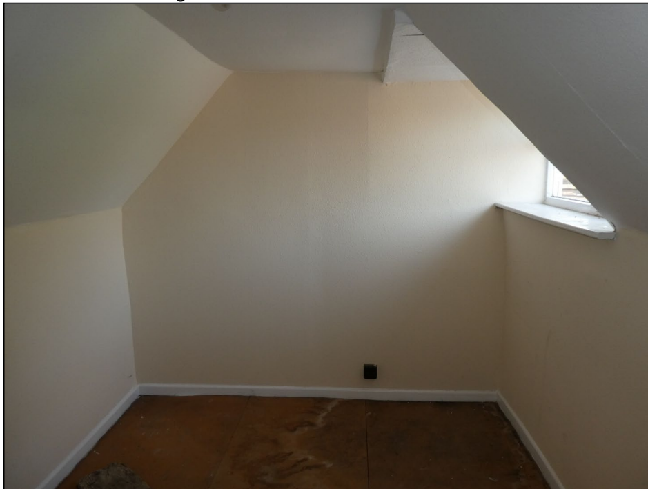
Figure 13. Example of internal habitable accommodation in former loft space. 36/38 Rose Street, Wokingham. RG40 1XU
