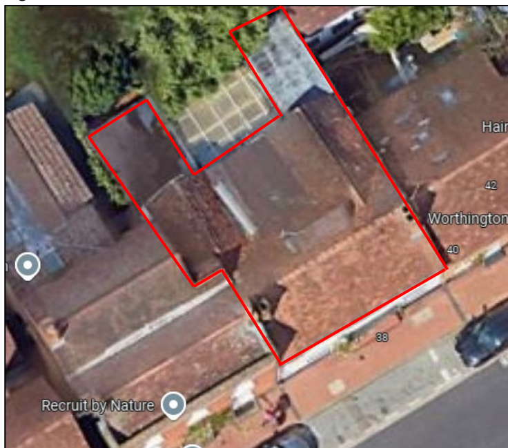
Figure 4. Roof structure outlined in red. 36/38 Rose Street, Wokingham. RG40 1XU
