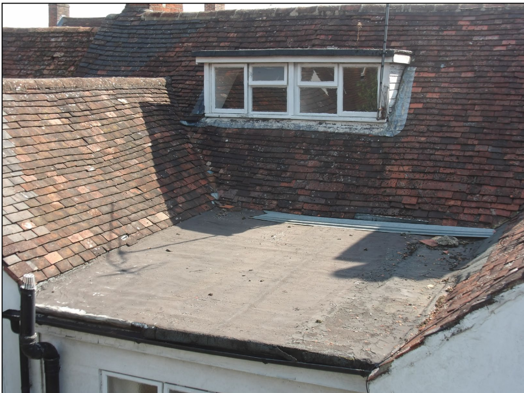
Figure 8. Rear flat roof at 1 st floor level. 36/38 Rose Street, Wokingham. RG40 1XU
