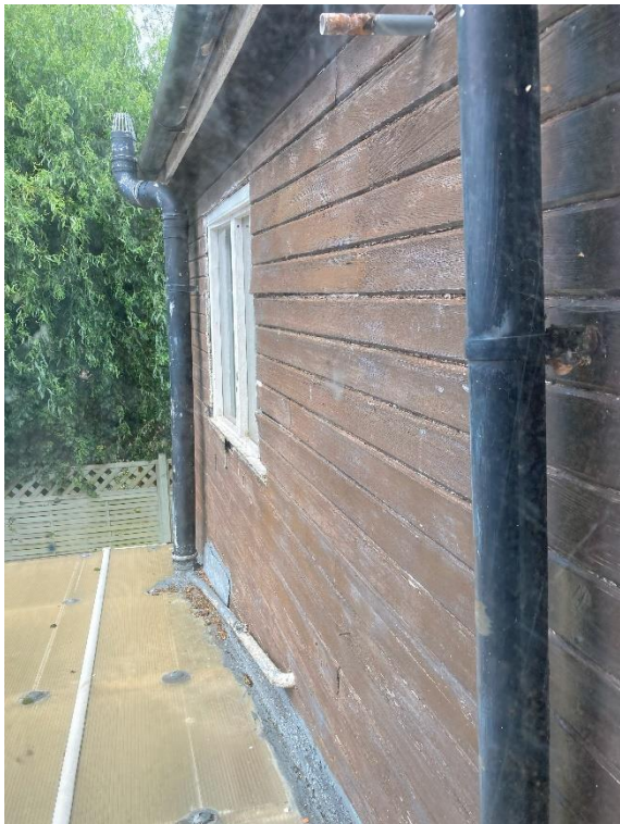
No.38 First Floor Extension
