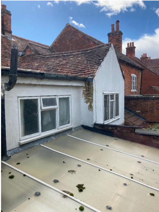
Conservatory roof with No.36 gable and flat roofing
