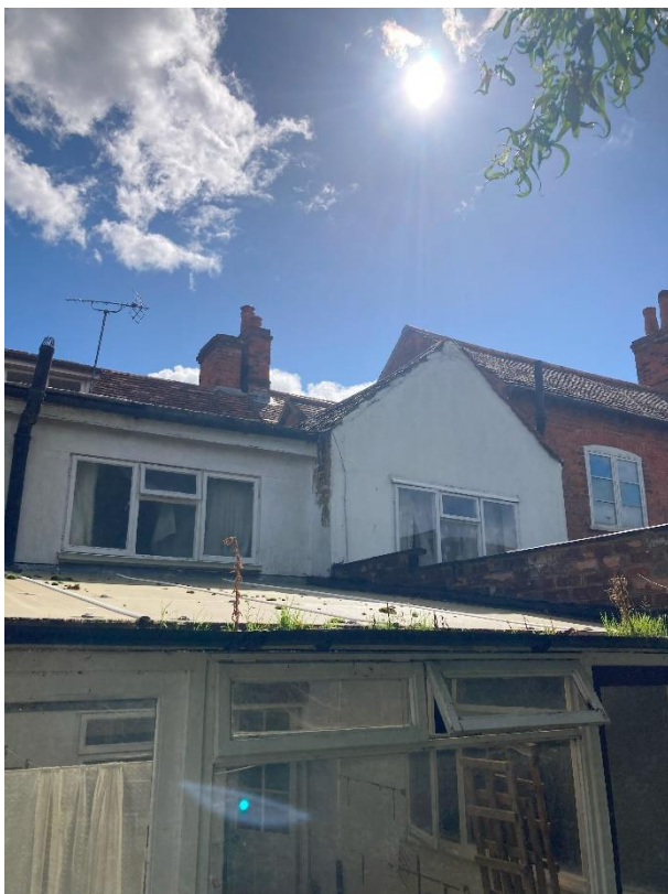
Gable end to No.36
