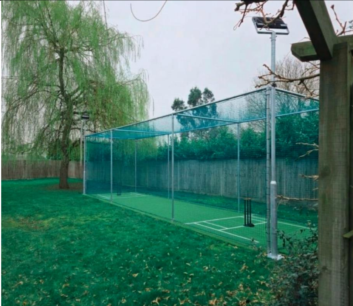
Visualisation of the proposed cricket practice pitch showing steel support poles, integrated LED floodlights, and protective cricket netting
