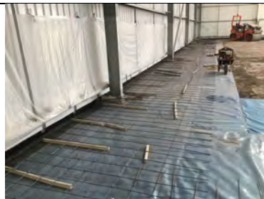
Overview of the Juta GP5 gas membrane installation as the pour progresses.
