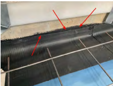
Evidence that the perimeter edge cladding rail was primed.
