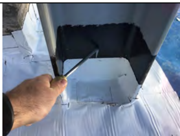
Probe testing all steel stanchion detailing in unit 1.
