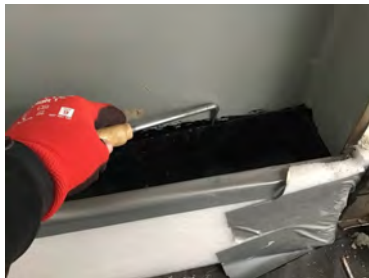
Probe testing all steel stanchion detailing.
