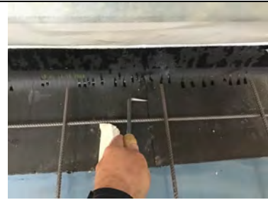
Probe testing the perimeter cladding rail detailing.
