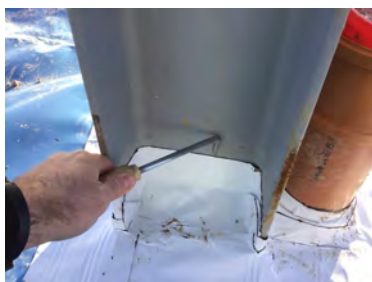
Probe testing all steel stanchions in unit 3.
