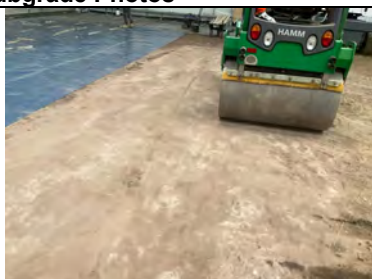
Substrate base being continuously rolled prior to gas membrane installation.
