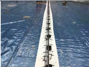
A strip of Juta GP SAM has been heat sealed to the Juta GP5 gas membrane across the armoured joint due to excessive holes found in the membrane due to follow on trades.
