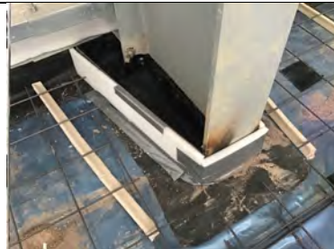
Steel stanchion detailing wrapped with miothene.
