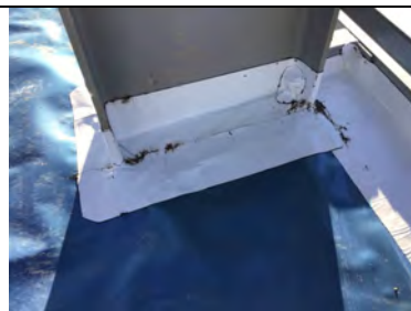
Steel stanchion detailing work in unit 2.
