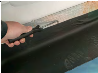
Probe testing along perimeter edge termination detailing.
