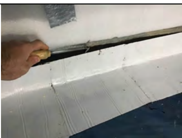
Probe testing the cladding rail detailing.
