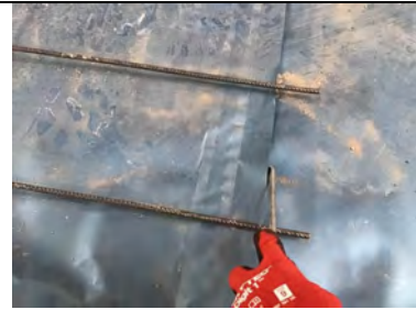
Probe testing an auto welded membrane lap.
