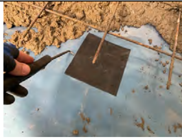
Defect was patched repaired using Juta GP1 SAM and probe tested.
