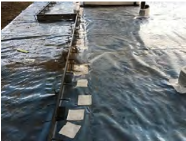
Patch repairs to damaged membrane along side the armoured joint pins in unit 7.
