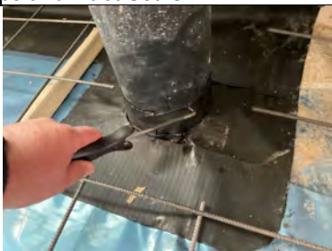
Probe testing to pipe penetration details.
