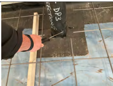
Probe testing to pipe penetration details.
