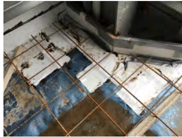
Overview of the patch repairs that have been achieved to the damaged membrane caused by follow on trades in unit 5 stair core area.
