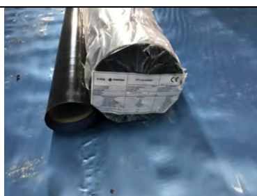
Evidence of the Juta GP5 gas membrane that has been installed as a full line out in unit 10.
