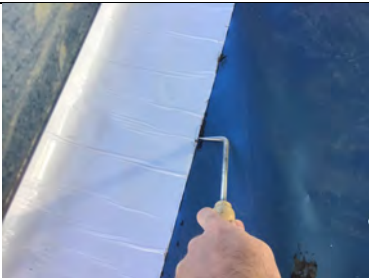
Probe testing the perimeter detailing work in unit 1.
