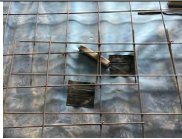
UK Membranes carried out the own CQA repairs as the pour progressed.
