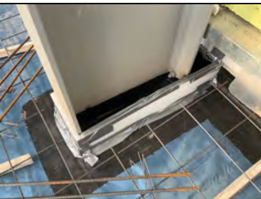
Steel stanchion detailed using Juta GP1 SAM but restricted inspection.
