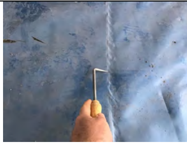
Probe testing all hand welded membrane laps.
