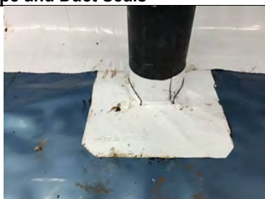
Typical pipe penetration detailing.
