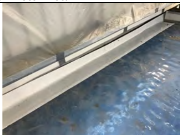
Retro fit detailing to the perimeter cladding rail.
