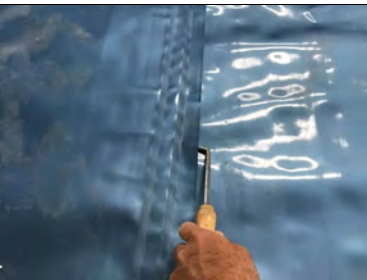
Probe testing all auto welded membrane laps.
