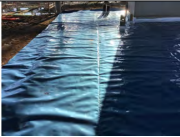
A typical hand welded membrane lap in unit 1.
