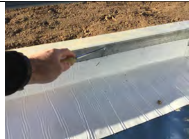
Probe testing the perimeter detailing work in units 2 & 3.
