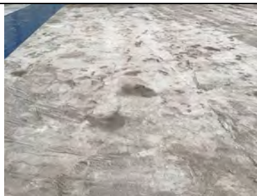
Evidence of a well rolled substrate.
