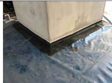
Retro fit detailing using Juta GP1 SAM around the corner lift pit.
