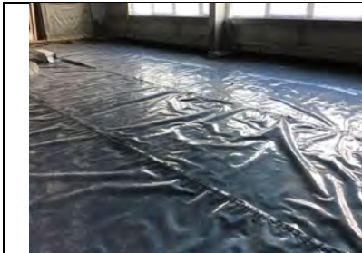
Overview of the Installed Juta GP5 gas membrane to the undercroft area in unit 2. ( marked in yellow on the site plan ).
