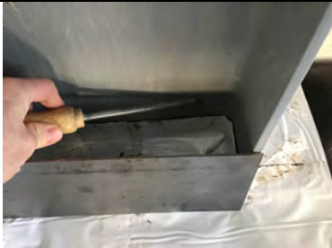
Probe testing the inner web of the stanchion detailing work.
