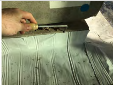
Probe testing to the stair core detailing.
