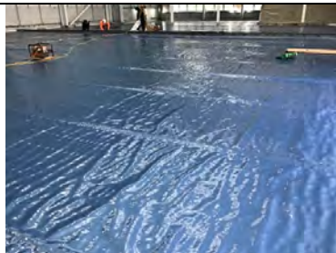
An overview of the Juta GP5 gas membrane that has been installed across the full footprint of unit 10.
