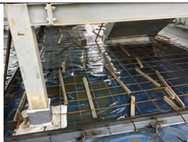
An overview of the Juta GP5 gas membrane installed to the stair core area in unit 4.
