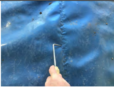
Probe testing all hand welded membrane laps.
