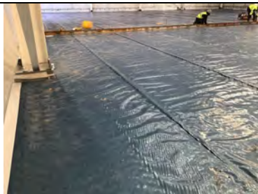
An overview of the Juta GP5 gas membrane that has been installed across the full footprint of unit 9.
