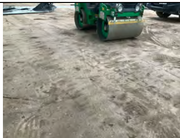
Substrate rolled in prep for gas membrane installation.
