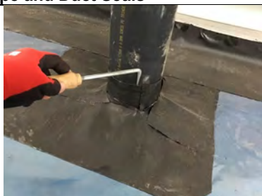
Probe testing a typical pipe penetration detail.
