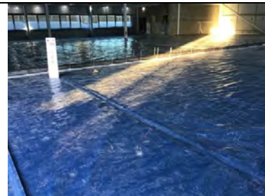
Overview of the Juta GP5 gas membrane that has been installed across the full footprint of unit 9.
