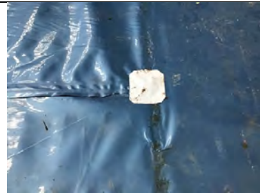
Patch repair using Juta GP SAM to a weld defect found upon our inspection.
