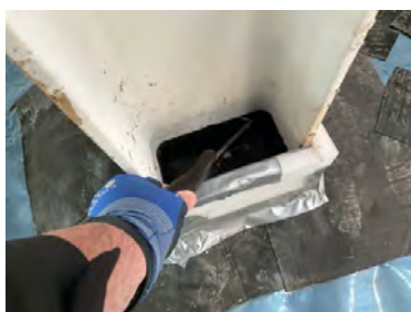
Probe testing to steel stanchion details.
