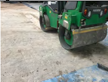
Evidence of the substrate being rolled prior to the installation of the Juta GP5 gas membrane as the pour progresses.
