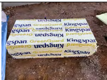
Evidence of the insulation boards used KingSpan GreenGuard.
