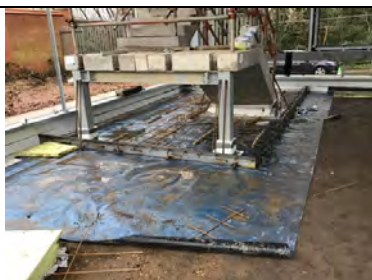
An overview of the Juta GP5 gas membrane installed to the stair core area in unit 5.
