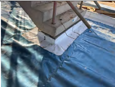
Stair Core. Base of the stair core was sealed using Juta GPSAM.
