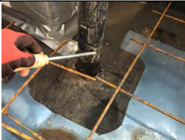
Probe testing a typical pipe penetration detail.
