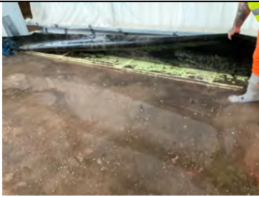
Flooding along perimeter edge.
