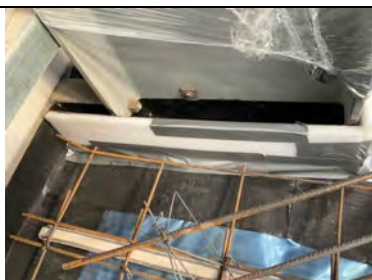
Restricted inspection to steel stanchion.
