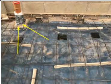
The pipe penetration was covered with miothene at the time of our inspection.
