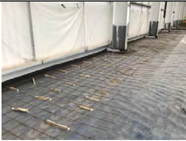
Overview of the Juta GP5 gas membrane around the perimeter of unit 8 with the steel mesh in place.
