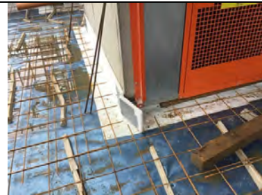
Miothene was covering the detailing work around the lift pit at the time of our inspection.
