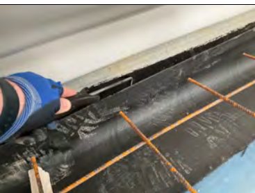
Probe testing along the perimeter edge cladding rail termination detailing
