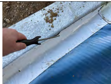
Entrance Lobby. Probe testing along the perimeter cladding rail termination.
