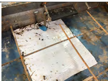
A patch of SAGM has been heat sealed to all damaged membrane around the armoured joint pins, sealing the base of the pins using double sided butyl tape.
