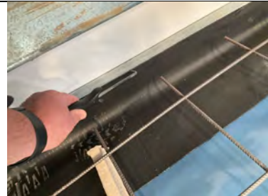
Probe testing along termination detailing to perimeter edge cladding rail.
