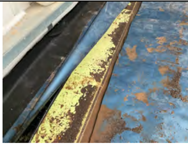
Membrane was cut to assess the existent of the water damage to substrate base.
