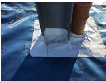
Typical steel stanchion detailing in unit 3.
