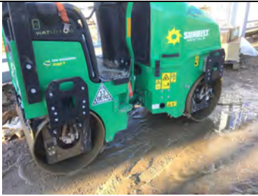
Evidence of the rolling machine that was used on the fine coarse aggregate substrate for the membrane to be laid upon.
