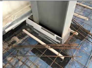
All steel stanchions were covered with miothene at the time of our inspection.
