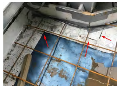
Slices in the membrane found upon our inspection.
