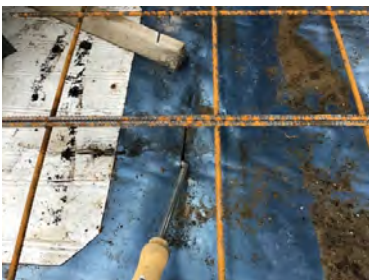
Slice in the membrane found upon our inspection.
