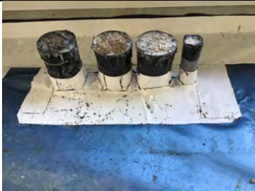
Typical pipe penetration detailing.
