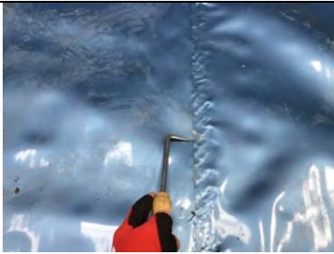
Probe testing all hand welded membrane laps.
