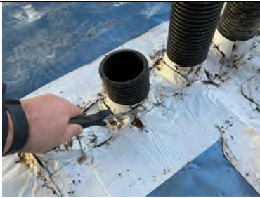
Entrance Lobby. Probe testing to sealed pipe penetration's.
