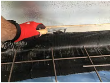
Probe testing the perimeter retro fit detailing.
