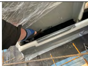
Probe testing to steel stanchion details.
