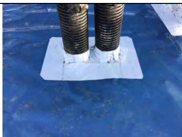
Typical pipe penetration detailing in unit 1.
