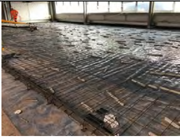
Overview of the Juta GP5 gas membrane installation to the undercroft in unit 8.
