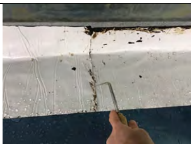
Probe testing all retro fit detailing in unit 4.
