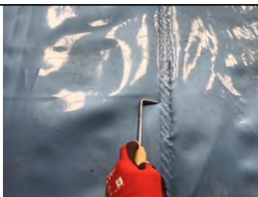
Probe testing all hand welded membrane laps.
