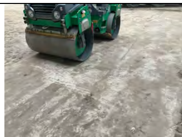
Substrate base being continuously rolled.
