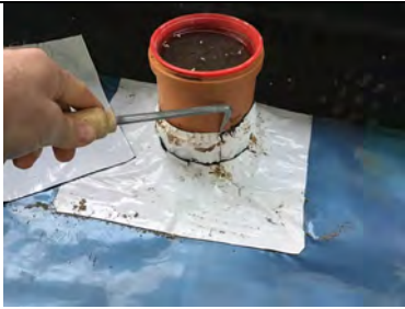
Probe testing all pipe penetration detailing.
