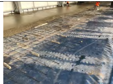
Overview of the Juta GP5 gas membrane installed on a just in time basis as the pour progresses.
