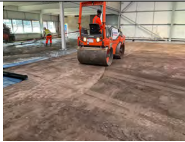
Substrate being continuously rolled prior to Juta GP5 gas barrier installation.
