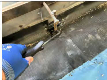
Probe testing to detailed armoured joint pins.
