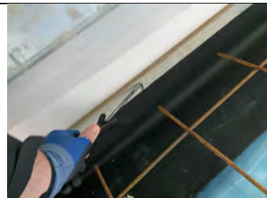
Probe testing to perimeter edge termination.
