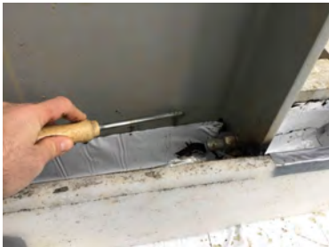
Probe testing to the inner web of the steel stanchion in unit 5.
