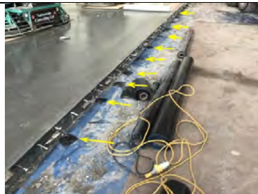
All armoured joint pin bases have been sealed using Juta GP1 SAM.
