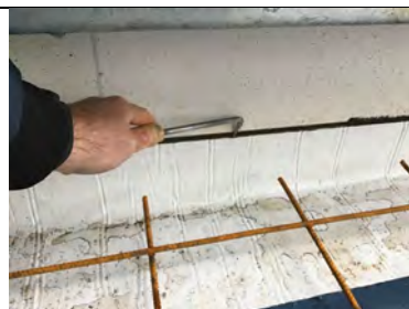
Probe testing the retro fit detailing in unit 5.
