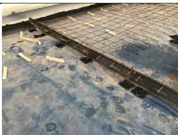
The armoured joint pin bases have been detailed using Juta GP1 SAM.
