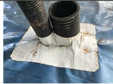
Typical pipe penetration detailing.
