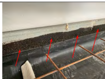
Evidence of the perimeter edge cladding rail being primed prior to termination detailing.
