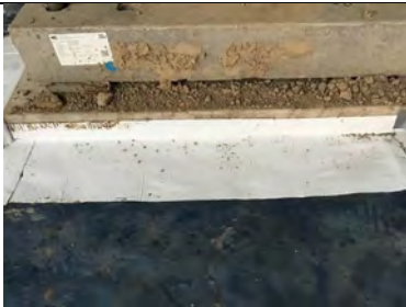
Retro fit detailing to the concrete stair core in unit 7.
