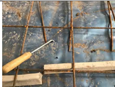
Damaged found in the membrane at the time of our inspection.
