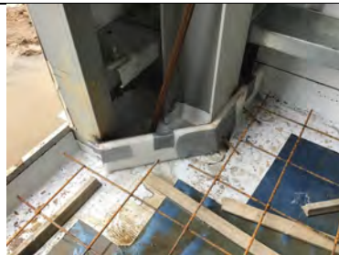
Restricted inspection to the detailing work around the steel stanchion in unit 4.
