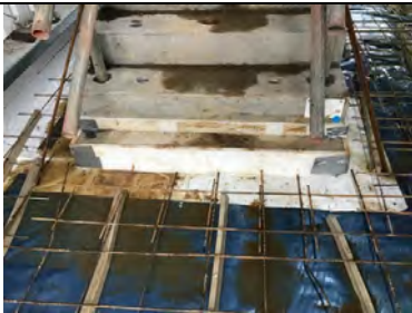
Restricted inspection to the bases of the concrete stairs due to the miothene in place.
