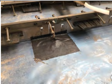
JUTA GP1 SAM wrapped around the armoured joint pins.
