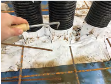
Probe testing all sealed pipe penetrations in unit 5 communal areas.
