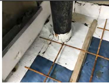
Typical pipe penetration detailing in unit 4.
