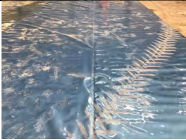
Overview of a typical hand welded membrane lap.
