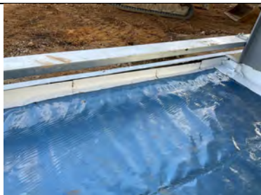
Entrance Lobby. Overview along the perimeter edge cladding rail sealed using Juta GPSAM.
