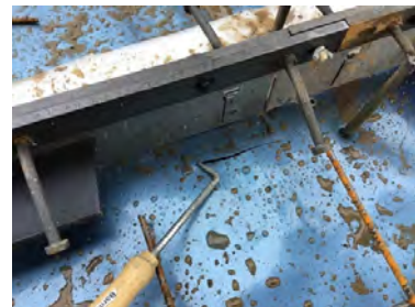
Damaged membrane was found upon our inspection.
