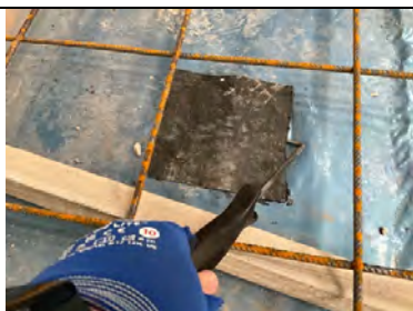
Probe testing installers own CQA patch repairs.
