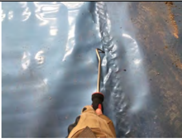
Testing to the hand welded lap joint.
