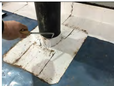
Probe testing a sealed pipe penetration.
