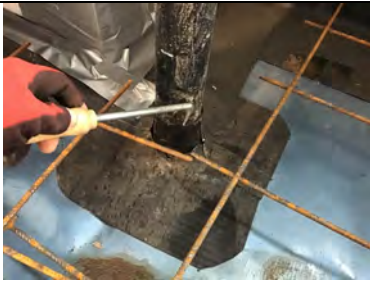
Probe testing a typical pipe penetration detail.
