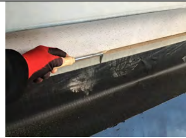
Probe testing all perimeter steel cladding rail retro fit detailing.
