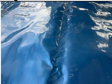
Entrance Lobby. Overview along a hand welded membrane lap joint.
