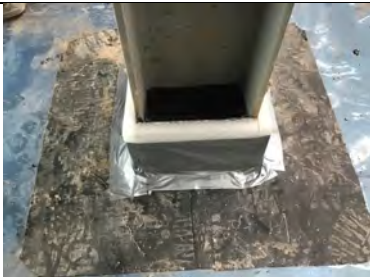
Restricted inspection of a steel stanchion due to the being wrapped in miothene.
