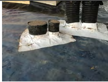
Typical pipe penetration detailing in unit 7 communal area.
