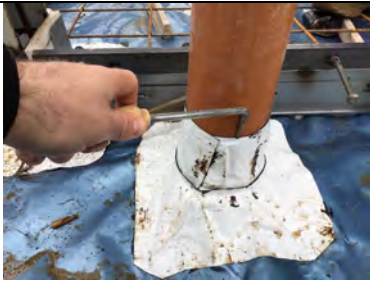
Probe testing a sealed pipe penetration in unit 4.
