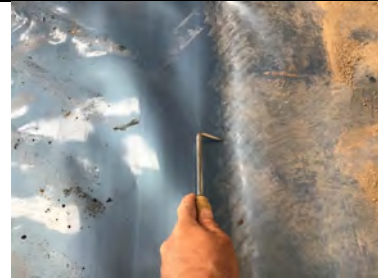
Probe testing a hand welded membrane lap.
