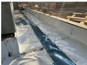
Stair Core. Overview along the perimeter edge cladding rail sealed using Juta GPSAM.
