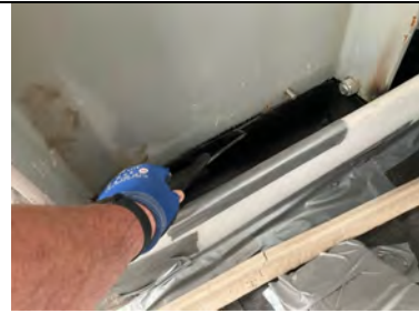
Probe testing to steel stanchion details.
