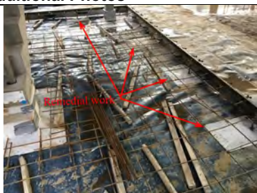
Overview of the remedial work that has been achieved by using SAGM around the armoured joint metal pins and using a strip of double sided butyl tape to the base of the pins in unit 4 stair core area.
