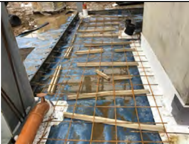
Miothene was in place around the lift pit detailing in units 4 & 5 at the time of our inspection.
