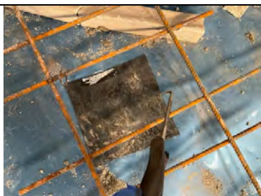
Recorded defect was patched repaired by installer using Juta GP1 SAM and probe tested.
