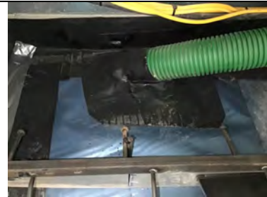
Typical pipe penetration detailing in unit 7.
