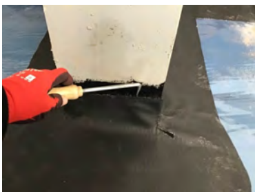
Probe testing a typical steel stanchion detail.
