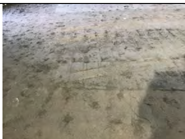
Evidence of a well rolled fine aggregate substrate that the membrane has been laid upon.
