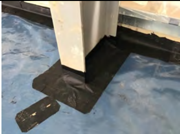
Typical steel stanchion detailing.
