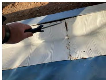
Stair Core. Probe testing along the perimeter cladding rail termination.
