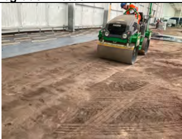
Substrate being continuously rolled prior to gas membrane installation.
