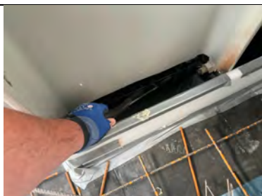
Probe testing to steel stanchion details.
