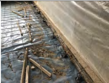
Armoured joint pin detailing using Juta GP1 SAM.
