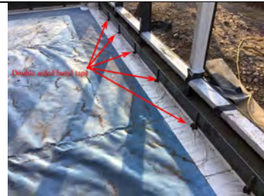
Double sided butyl tape used on the bases of the metal rods used for the armoured joints.
