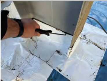
Entrance Lobby. Probe testing to sealed steel stanchions.
