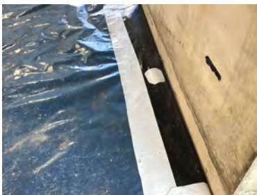
SAGM detailing to the extended membrane underneath the lift pit.
