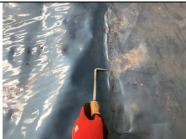
Probe testing the hand welded membrane lap.
