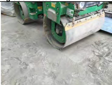
Evidence of the substrate being rolled prior to the installation of the Juta GP5 gas membrane as the pour progresses.
