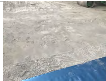
A well rolled fine coarse aggregate substrate.
