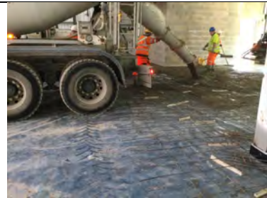
Concrete wagon kept off the steel mesh
