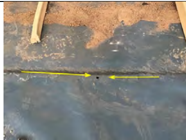
Hole found in the membrane during our inspection.
