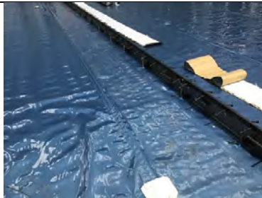
Double sided tape has been used to sealed the armoured joint metal pins.
