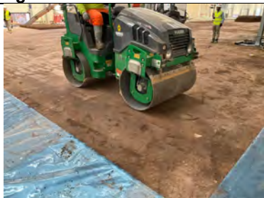
Substrate being continuously rolled.
