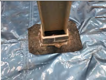
Steel stanchion wrapped in miothene during our inspection.
