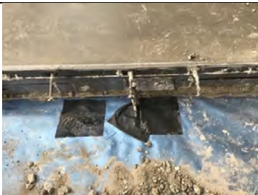
The bases of the armoured joint pin holes have been sealed using Juta GP1 SAM.
