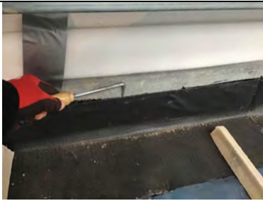
Probe test the perimeter retro fit detailing.
