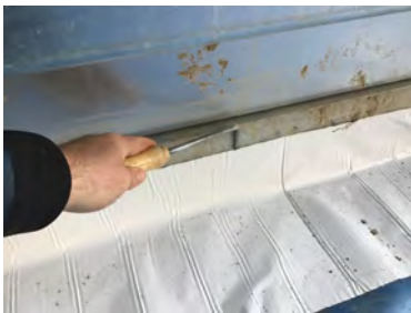
Probe testing all perimeter detailing within units 7 & 8.
