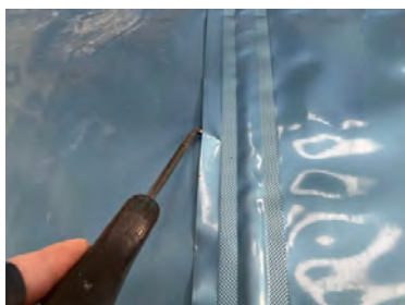
Probe testing along auto welded membrane lap joints.
