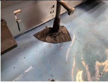
Armoured joint pins were detailed using Jute GP1 SAM.
