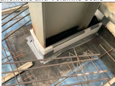
Restricted inspection to steel stanchions due to miothene strips surrounding.
