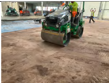
Substrate was well rolled prior to gas barrier installation.
