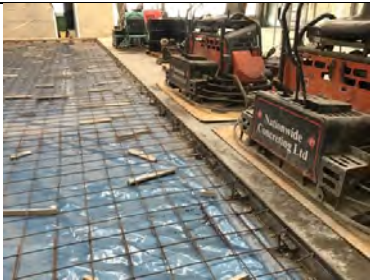
All armoured joint pin holes have been sealed using Juta GP1 SAM.
