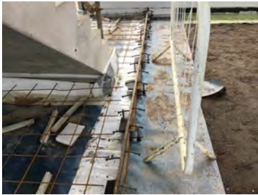
Retro fit detail using SAGM to all damaged areas in unit 5 stair core area.
