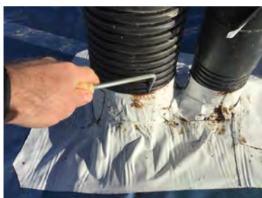
Probe testing all pipe penetration detailing in unit 3.
