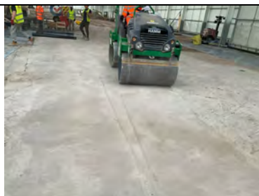
Substrate was continuously rolled.
