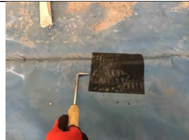
Probe testing the repaired hole found in the membrane.
