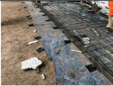
Armoured joint pin hole detailing.
