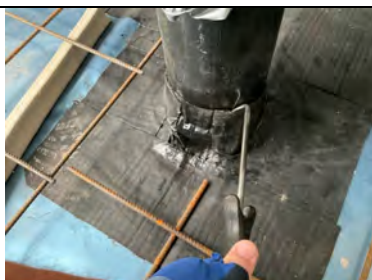
Probe testing to pipe penetration details.
