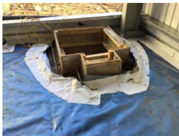
The SAGM has been sealed to the extended membrane that was previously installed underneath the service pit, the membrane underneath the service pit has not been inspected by MEC Environmental. I can therefore confirm that the membrane has been installed correctly.
