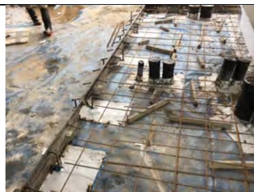
Overview of the remedial work that has been achieved by using SAGM around the armoured joint metal pins and using a strip of double sided butyl tape to the base of the pins in unit 4 communal area.
