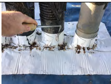
Probe testing all pipe penetration detailing in unit 1.
