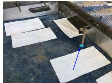
Double sided butyl tape has been used to seal the base of the armoured joint pins.
