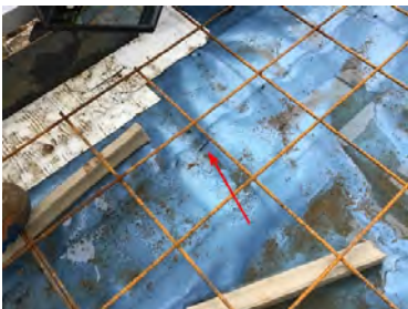
Damaged membrane was found during our inspection.
