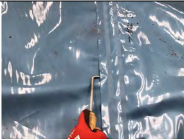
Probe testing all auto welded membrane laps.
