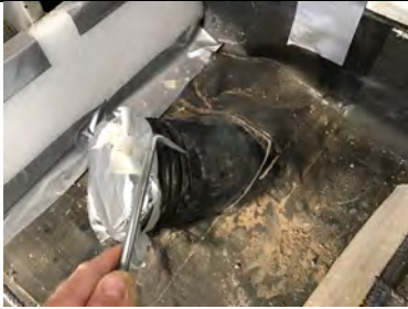
Probe testing a typical pipe penetration detail.
