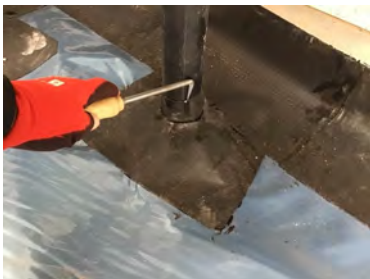
Probe testing a typical pipe penetration in unit 8.
