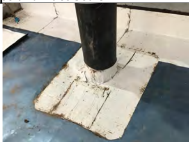
Typical pipe penetration detailing.
