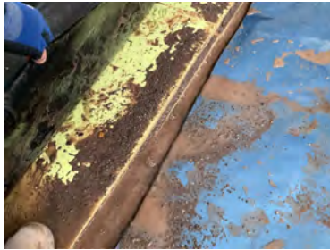
Insulation boards lifting due to the water damage along the perimeter edge and softening of the substrate base.
