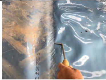
Probe testing all hand welded membrane laps.
