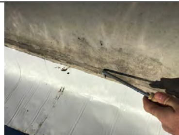
Probe testing the detailing work around the lift pit in unit 1.
