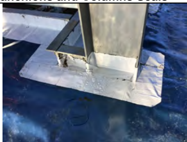
Typical stanchion detailing work in unit 1.
