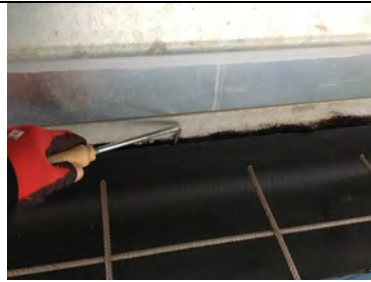
Probe testing the perimeter retro detailing.
