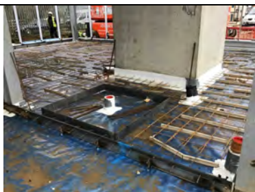
Overview of the Juta GP5 gas membrane that has been installed to the communal area in unit 5.
