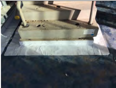
Retro fit detailing to the base of the concrete stair core.
