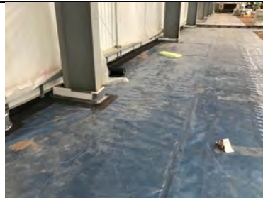
Overview of the Juta GP5 gas membrane installed to the perimeter edge in unit 2 ( marked in yellow on the site plan ).
