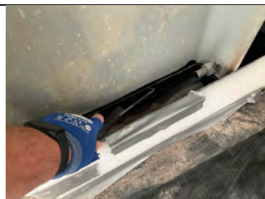
Probe testing to steel stanchion details.
