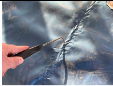
Stair Core. Probe testing along hand welded membrane lap joints.
