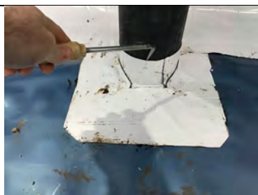
Probe testing the pipe penetration detailing.
