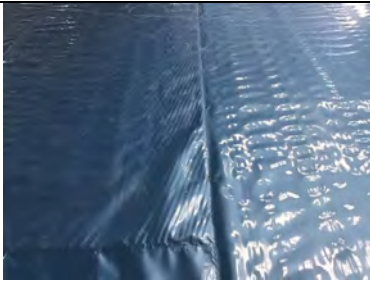
Overview of a typical hand welded membrane lap.
