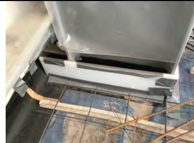
Miothene was in place around the steel stanchions at the time of our inspection.
