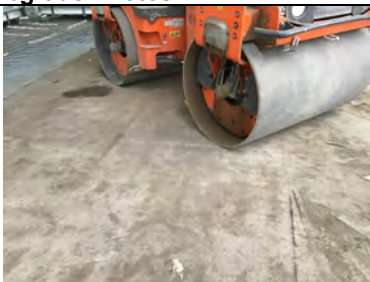
The substrate had been continuously rolled during the installation of the gas membrane as the pour progresses.
