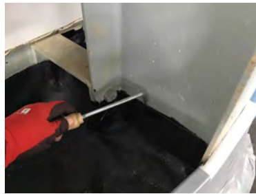
Probe testing the inner web of the steel stanchion.
