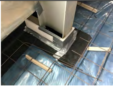
Steel stanchion detailing that has been covered with miothene prior to our inspection.
