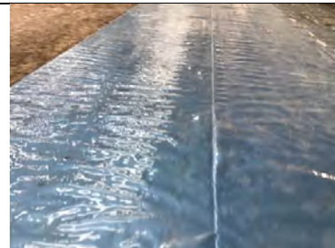
Typical hand welded membrane lap.
