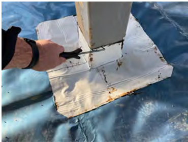
Stair Core. Probe testing to sealed steel stanchions.
