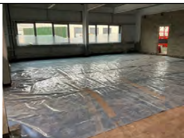
Overview of Unit 3 Undercroft full line out using Juta GP5 gas barrier.
