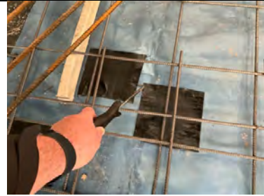
Probe testing to installer CQA patch repairs.
