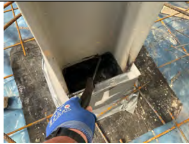
Probe testing to steel stanchion details.
