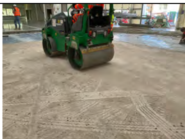
Substrate being rolled prior to gas barrier installation.
