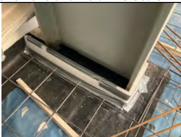
Steel stanchion detailed using Juta GP1 SAM but restricted inspection.
