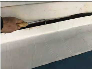
Probe testing all perimeter detailing.
