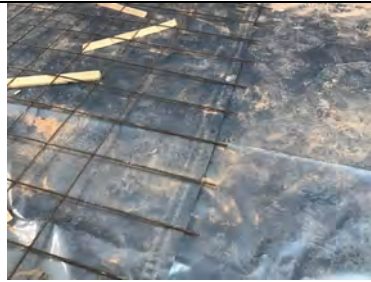
Overview of a auto welded membrane lap.
