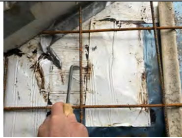
Probe testing all SAGM remedial work that has been done across units 4 & 5.
