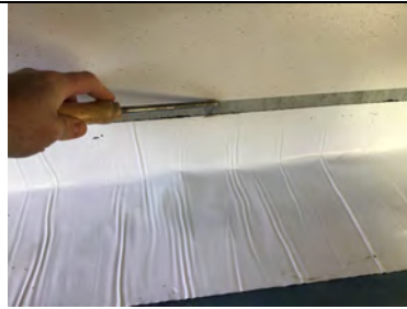
Probe testing all perimeter detailing work.
