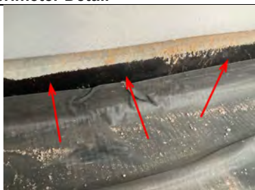
Evidence that the perimeter cladding rail was primed prior to termination detailing.
