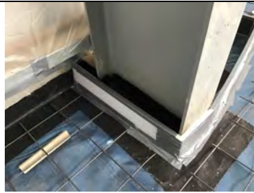
Steel stanchion detailing that has been wrapped with miothene.
