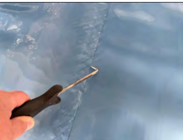
Probe testing along hand welded membrane lap joints.
