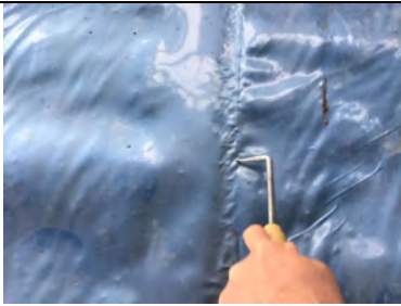
Probe testing all typical hand welded membrane laps.
