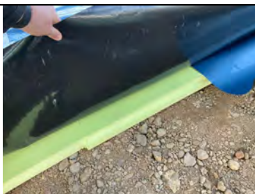
Evidence of KingSpan GreenGuard below gas barrier.
