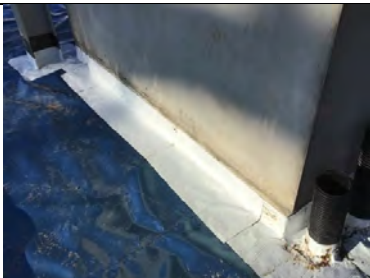
Retro fit detailing to the precast concrete lift pit wall in unit 1.
