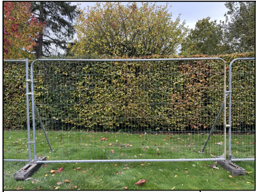
Protective Barrier (P.B.) Standard Tree Protection (S.T.P.) Heras fencing panels.
