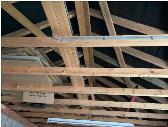
Photograph 12. Trussed roof with bitumen reinforced liner.
