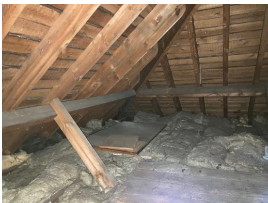
Photograph 9. Roof void with timber sarking lining.
