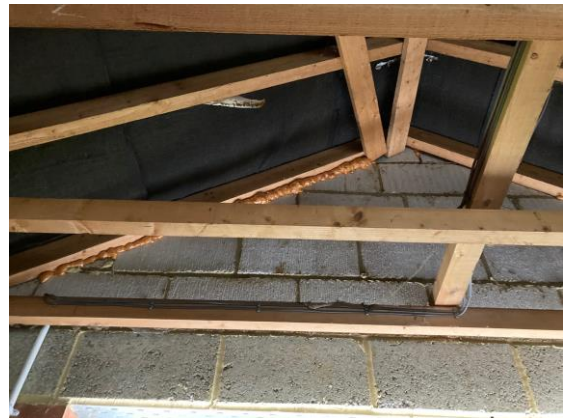
Photograph 13. Expanding foam between end rafter and blockwork gable.
