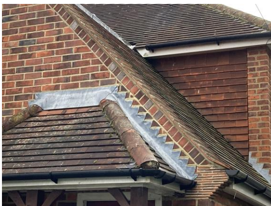
Photograph 7. Flat and tight hanging tiles.
