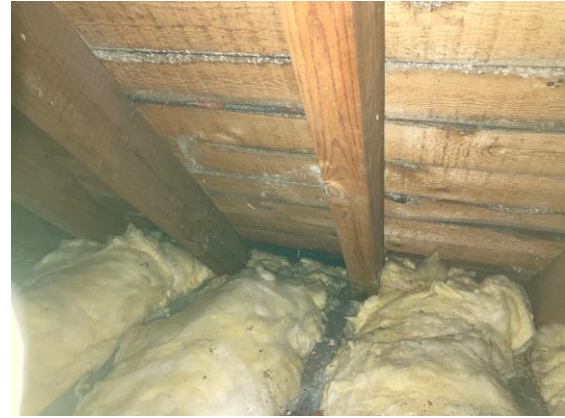
Photograph 12. Eaves filled with fibreglass insulation.
