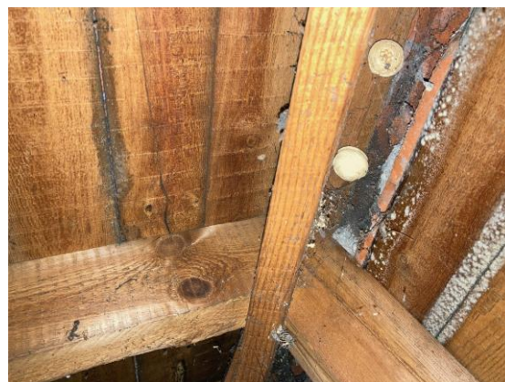
Photograph 10. Roof tiles visible at top of sarking up to ridge beam.
