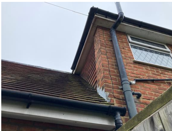
Photograph 5. Soffits tight throughout.
