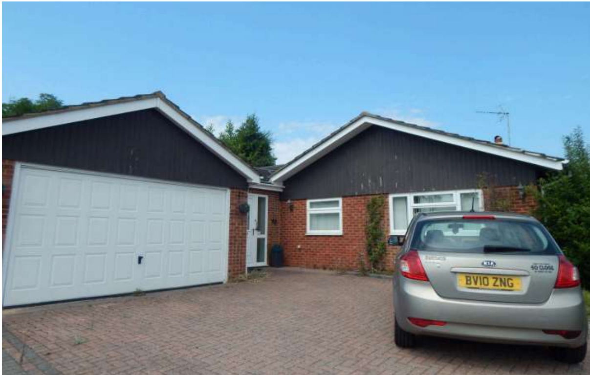
Image 1 – South facing elevation of the main dwellings and East facing elevation of the garage section
