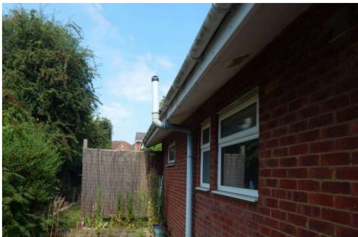
Image 4 – East facing elevation of the dwelling
