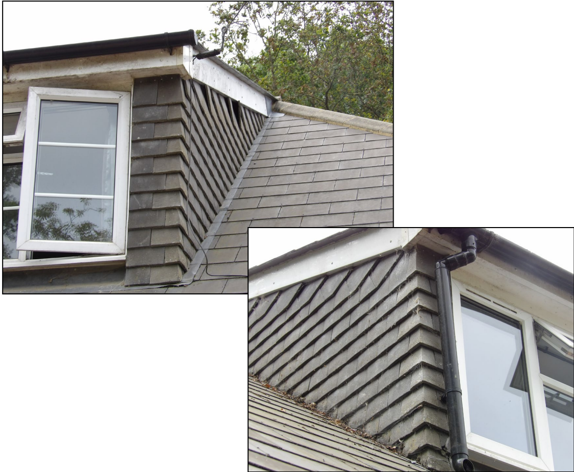
Figure 9. Example well fitted soffits/fascias. Willow Tree House, Wokingham. 19.08.25
