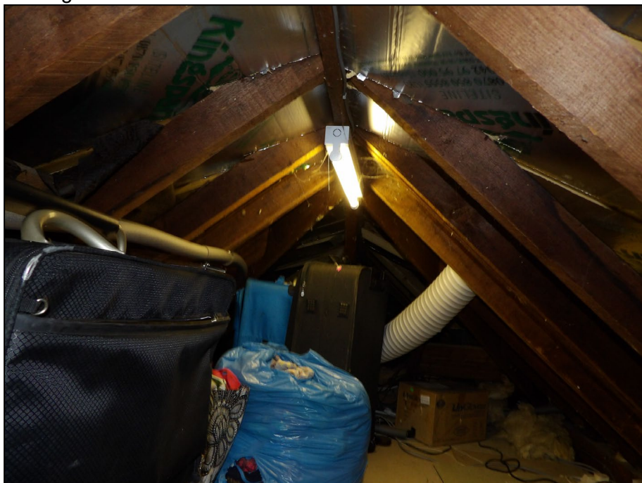
Figure 10. Loft space and Kingspan insulation to roof tiles. Willow Tree House, Wokingham. 19.08.25
