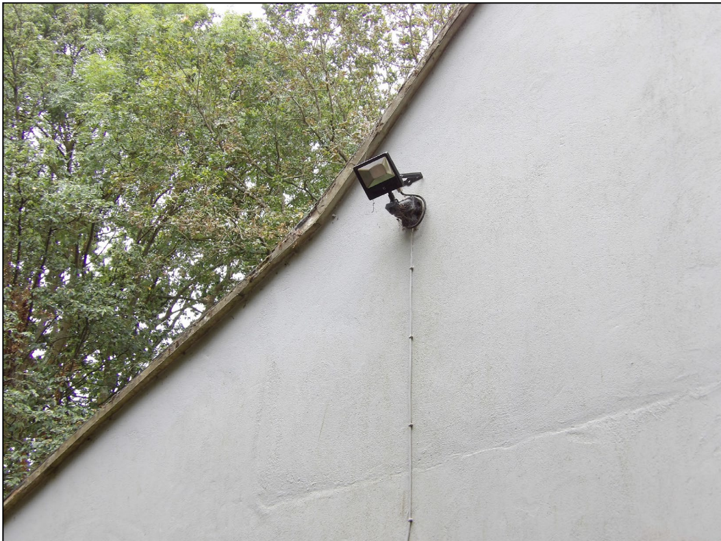
Figure 7. Example sealed verges. Willow Tree House, Wokingham. 19.08.25
