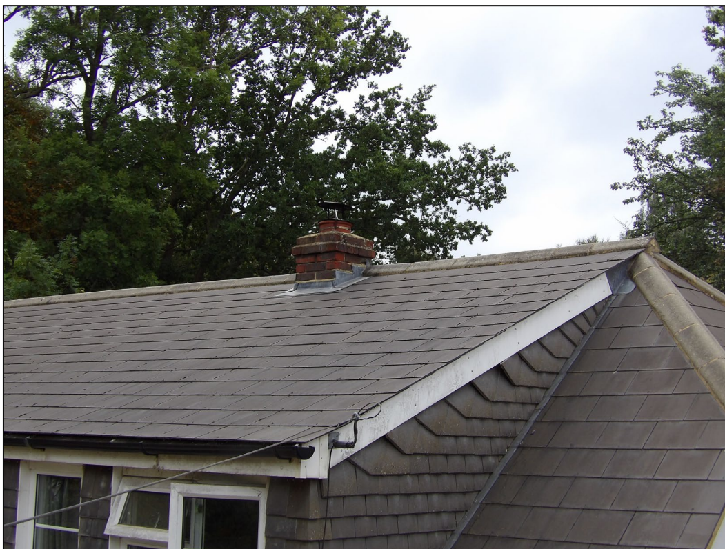
Figure 5. Example sealed roof/ridge and hip tiles. Willow Tree House, Wokingham. 19.08.25
