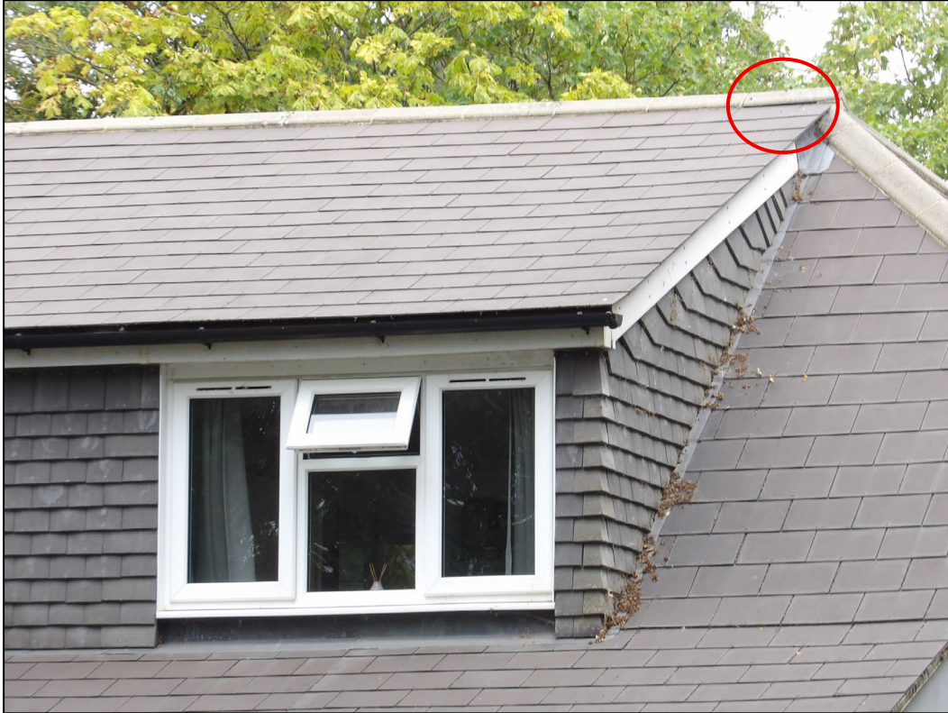
Figure 6. Missing mortar from ridge tiles on rear elevation. Willow Tree House, Wokingham. 19.08.25
