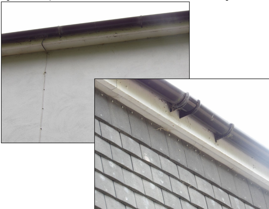
Figure 9. Example well fitted soffits/fascias. Willow Tree House, Wokingham. 19.08.25
