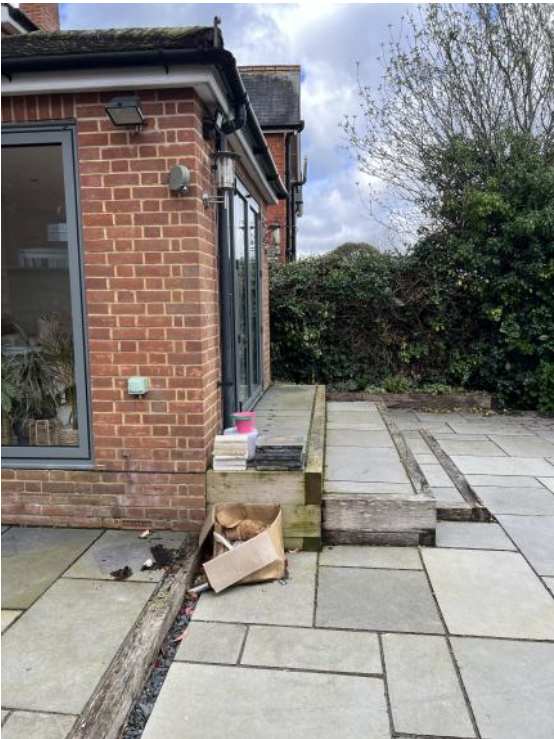
View towards adjoining
