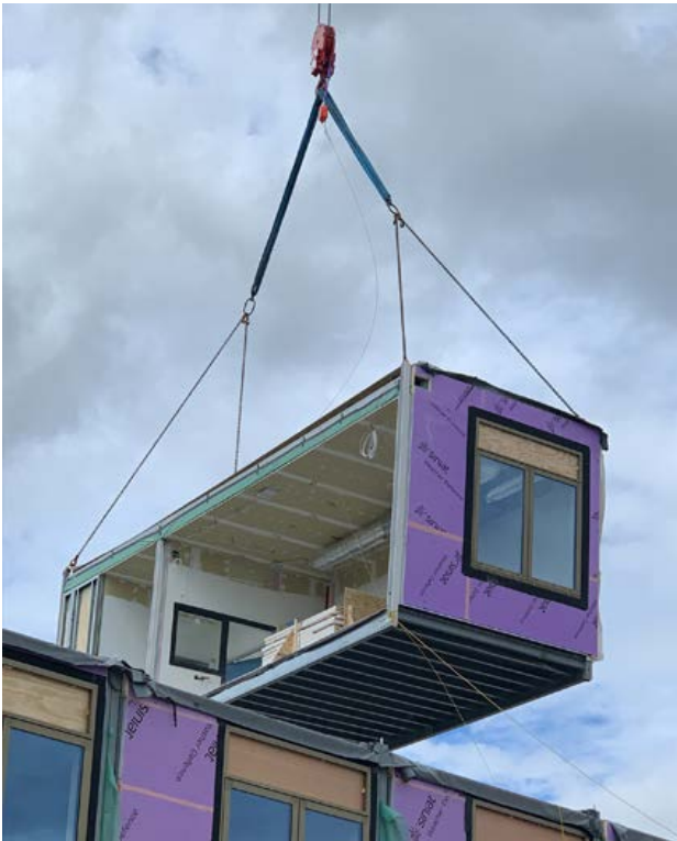
Example of modular unit being installed by crane
