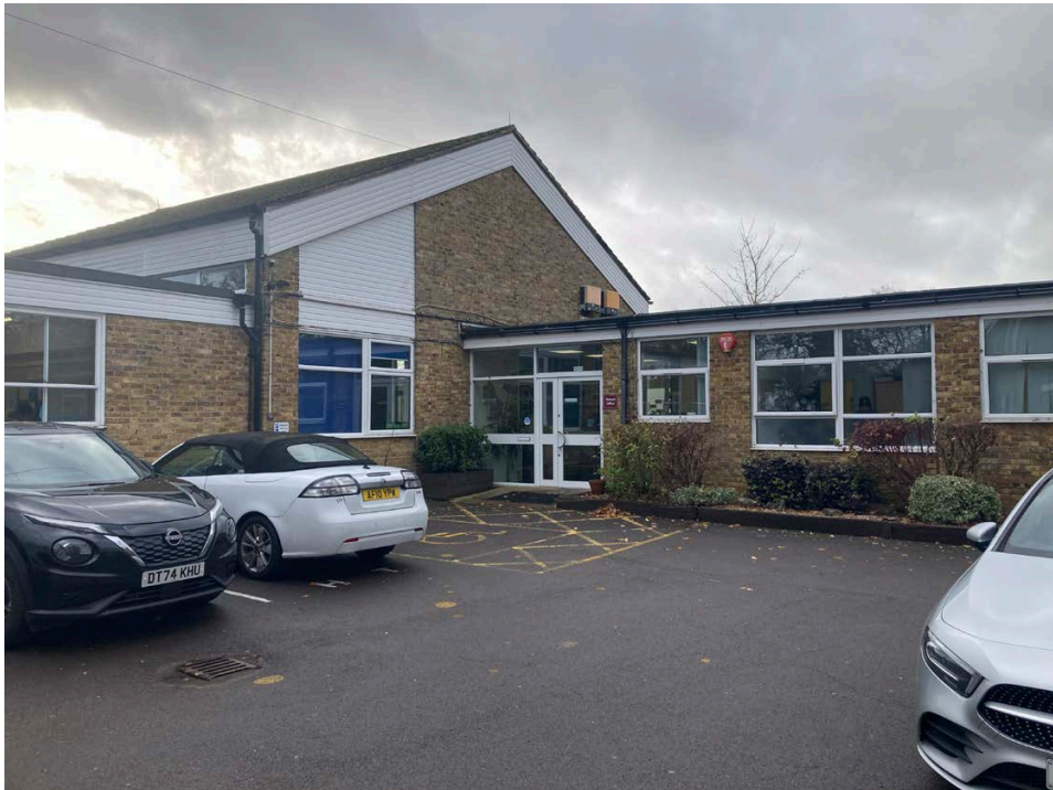
Main entrance for visitors
