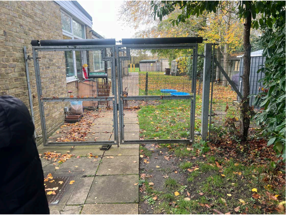
Gated maintenance access to north west of school
