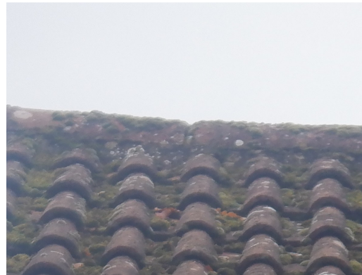
Photograph 4. Intact ridge mortar (front elevation).
