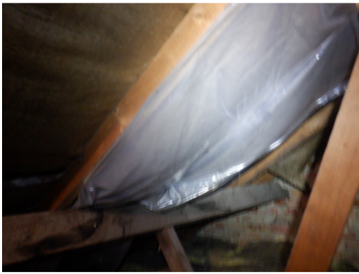
Photograph 11. Section of roof on eastern side of roof void that is lined with plastic sheeting (roof void).
