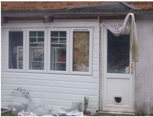
Photograph 7. Rear extension with bitumen felt flat roof and uPVC boarding (rear elevation).
