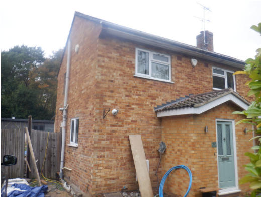
Photograph 1. Front of house viewed from southwest.
