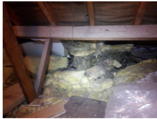
Photograph 12. Thick fibreglass between joists on floor of roof void (roof void).
