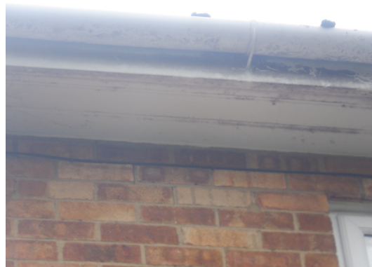
Photograph 6. Intact soffits and fascias tight to the brick of the property (front elevation).
