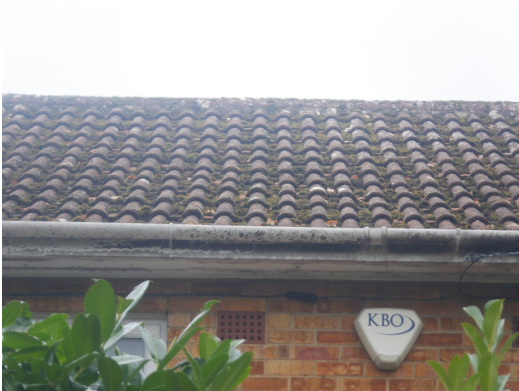
Photograph 3. Intact/tight interlocking roof tiles (front elevation).
