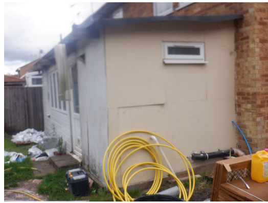
Photograph 8. Chipboard construction of rear extension (eastern elevation).
