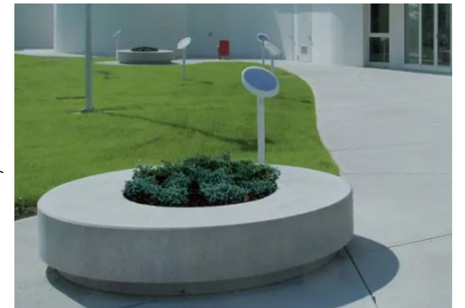
Round concrete benches with planting in the centre anchor the edges of the wet pour surface and provide informal seating and further playful edges for children to climb on.
