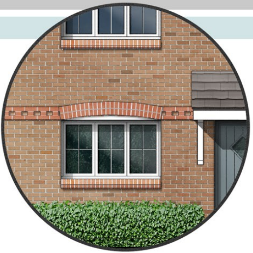
Brick Dental Course in Contrasting Brickwork to selected plots
