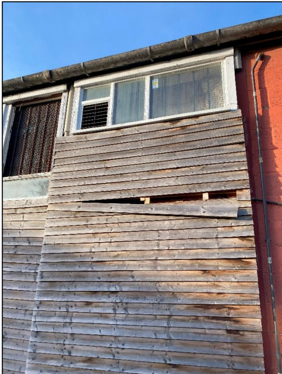
Image 2: Slipped wooden boards on B2
