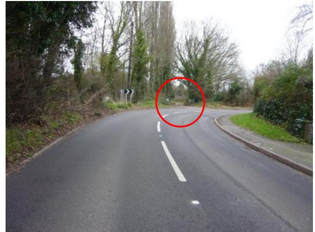
View looking east towards private road / bridleway.
