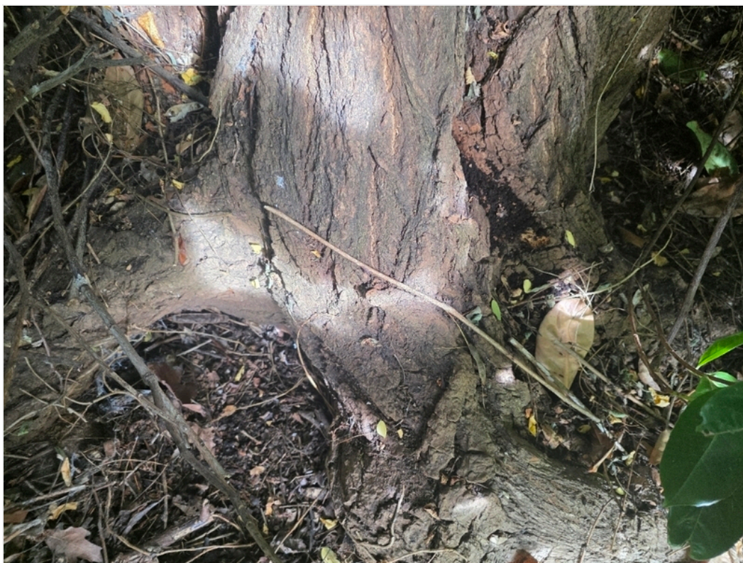
T01 - Cavity at base (no decay detected)
