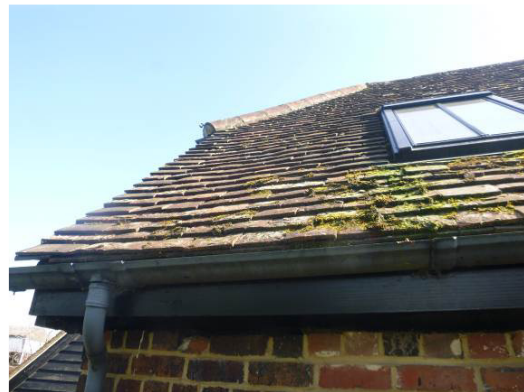
Photograph 5. Handmade clay tiles (western elevation).
