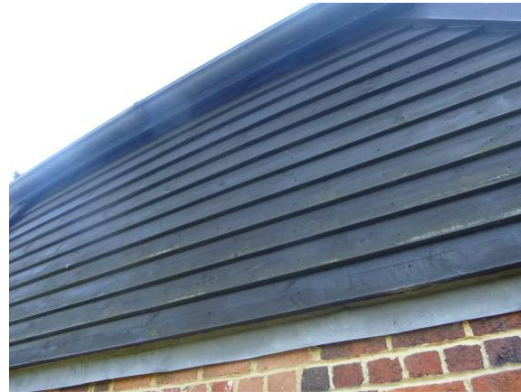
Photograph 7. Western gable (western elevation).
