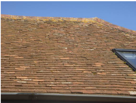
Photograph 4. Handmade clay tiles (front elevation).
