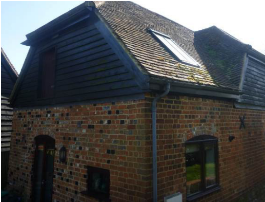
Photograph 3. Rear of property viewed from north.
