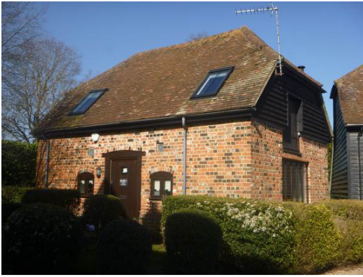
Photograph 1. Front of property viewed from south.
