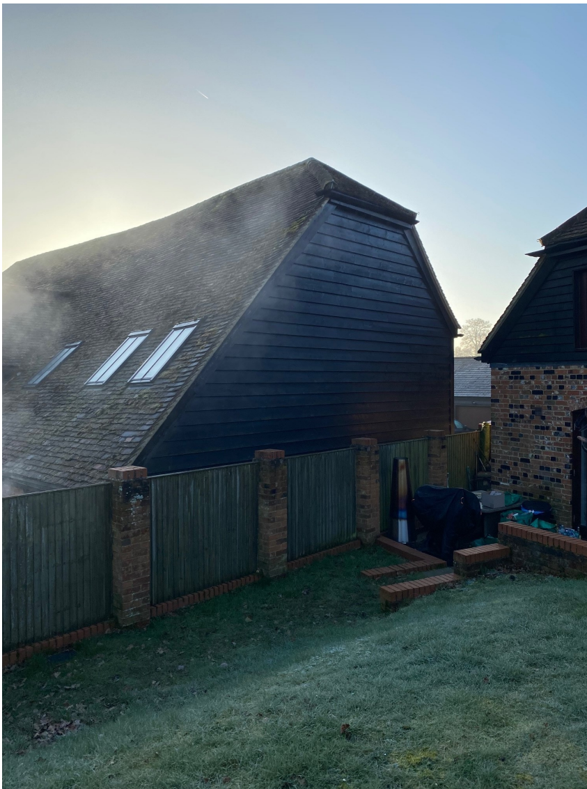
PIC 6. VIEW FROM GARDEN OF BARN 1
