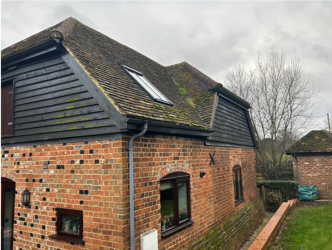
PIC 5. EXISTING SIDE ELEVATION SHOWING WHERE THE EXTENSION WILL BE ADDED
