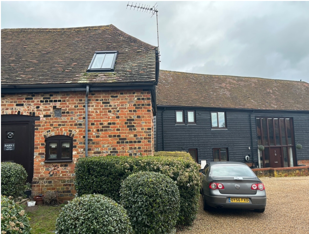
PIC 2. EXISTING FRONT ELEVATION SHOWING BARN 2
