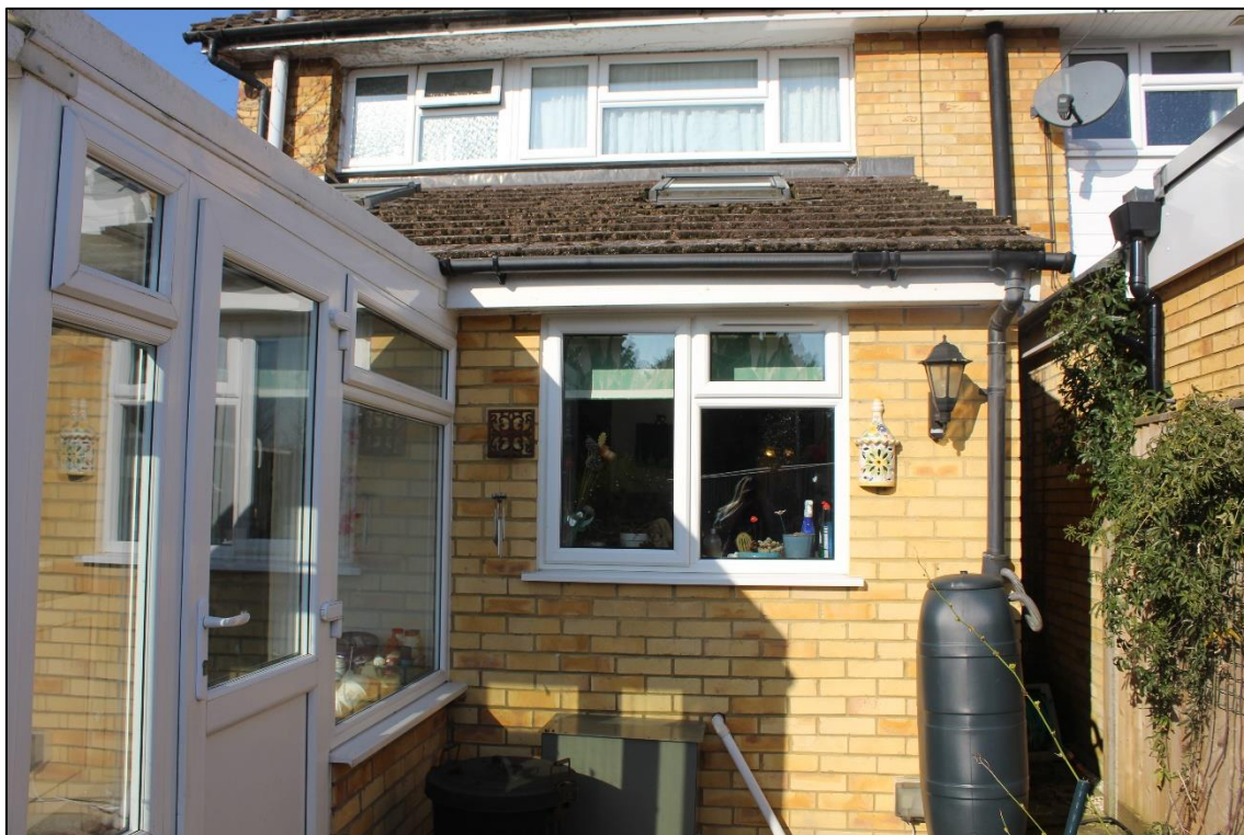
Photograph 2 – Rear elevation showing single-storey rear extension and existing conservatory
