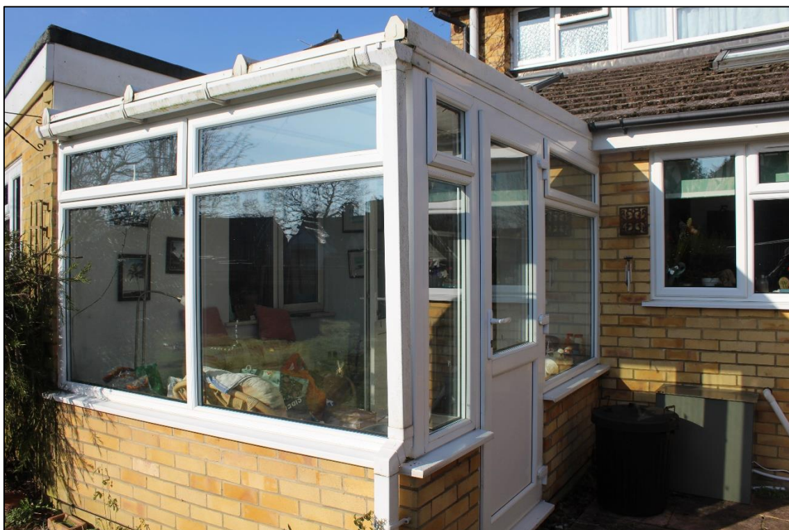
Photograph 3 – Rear elevation showing the existing conservatory
