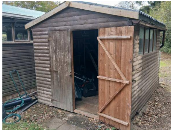
Eastern elevation of building B2.
