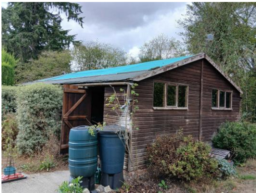
Northern elevation of B1.
