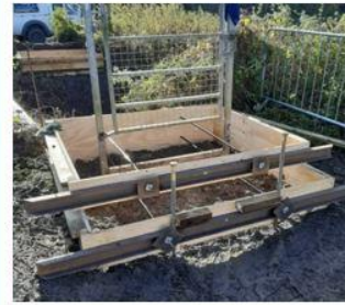
Concrete cast in situ
