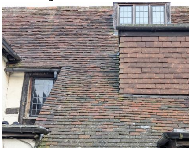
Photograph 4: Hanging tiles on dormer on north pitch
