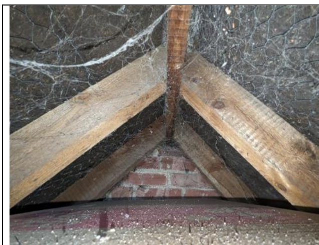
Photograph 3: Heavily cobwebbed ridge of eastern side of main void
