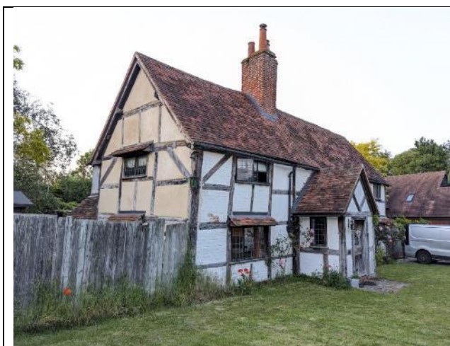
Photograph 1: South and west elevations and example of awnings
