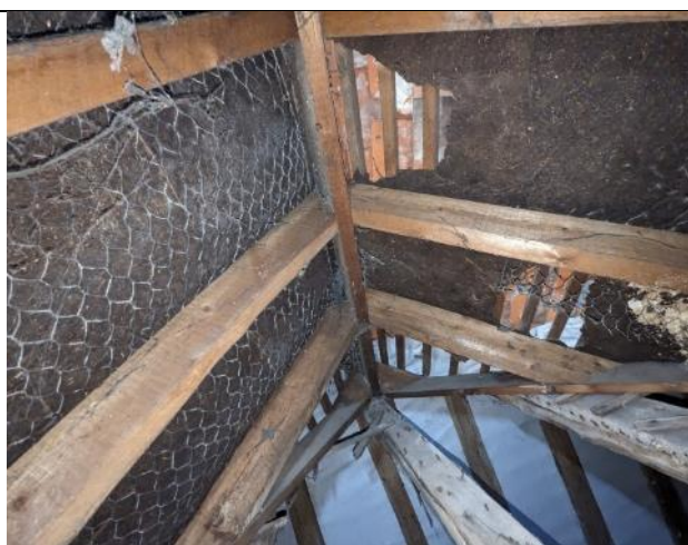
Photograph 4: Chicken wire-lined pitch of western-side of main void
