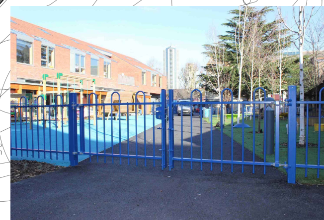
Low Level Fencing
