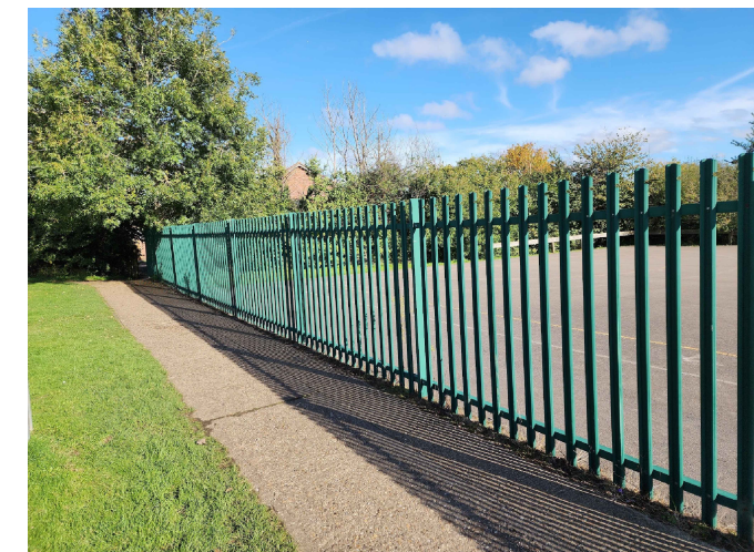
Existing Palisade Fencing
