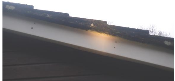
Photograph 7. Verge mortar fully intact (rear elevation).
