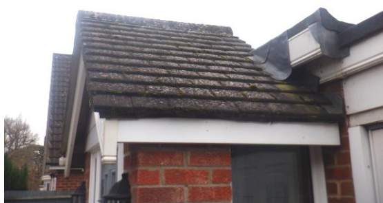
Photograph 4. Sealed clay roof tiles (east elevation).
