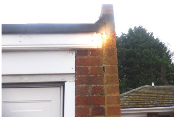
Photograph 5. Sealed bitumen felt (front elevation).
