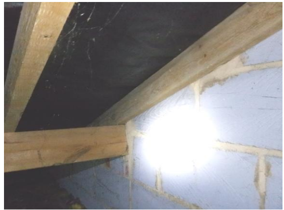
Photograph 20. Timbers sealed to front blockwork gable.
