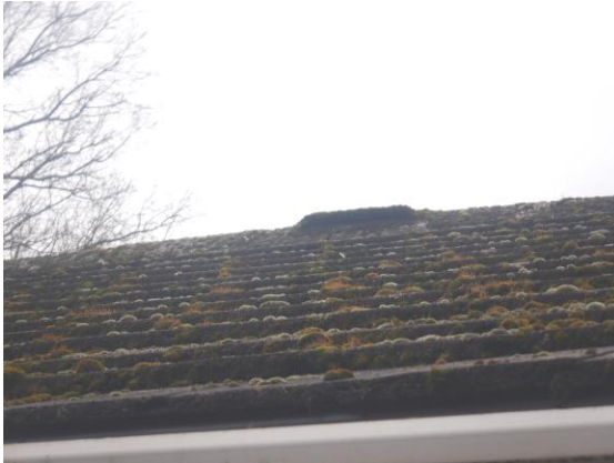
Photograph 6. Ridge mortar intact (east elevation).
