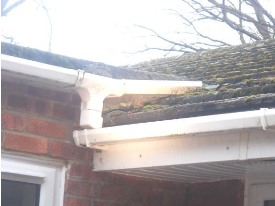
Photograph 12. Junction between flat roof and pitched roof fully sealed (east elevation).
