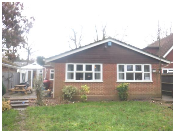
Photograph 2. Rear elevation of the property, viewed from the north.
