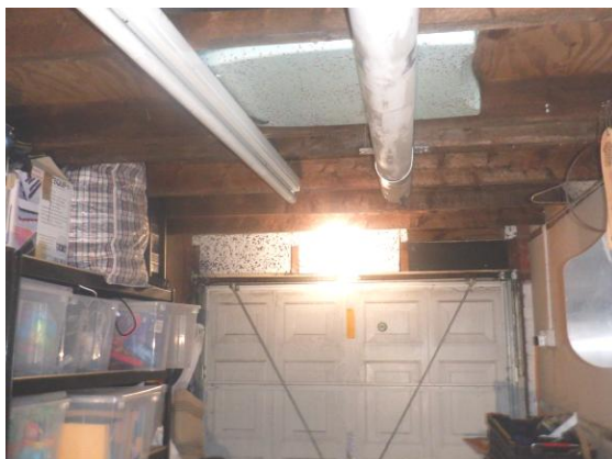
Photograph 23. Garage with boarded ceiling sealed to polystyrene panels.
