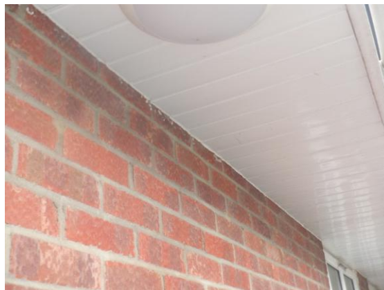
Photograph 16. uPVC soffit sealed to brickwork wall (west elevation).
