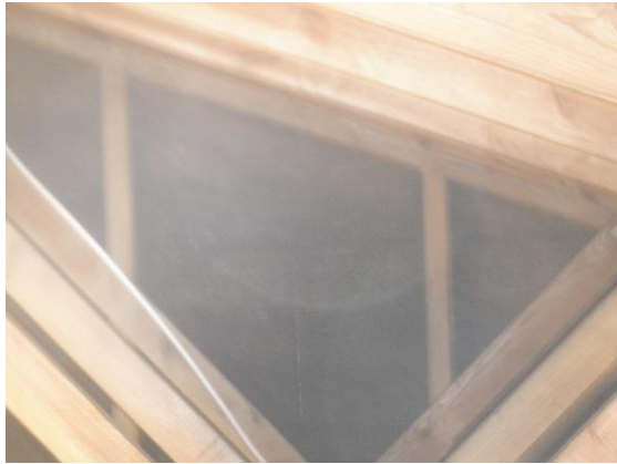
Photograph 21. Rear gable clad with bitumen felt and sealed to timbers.
