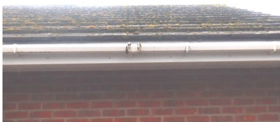
Photograph 3. Flat concrete roof tiles (east elevation).
