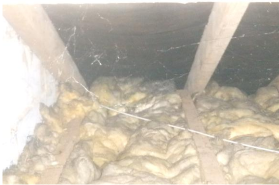
Photograph 19. Open eaves with access to the uPVC soffit.
