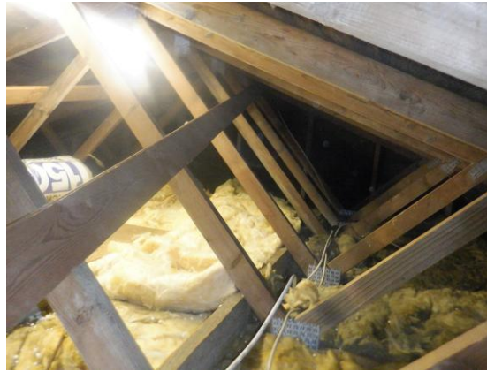
Photograph 17. Void of trussed construction.
