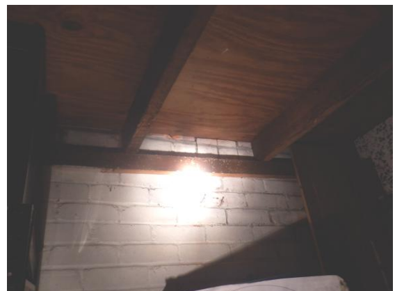
Photograph 24. Timber panels sealed to the painted brickwork walls (garage).
