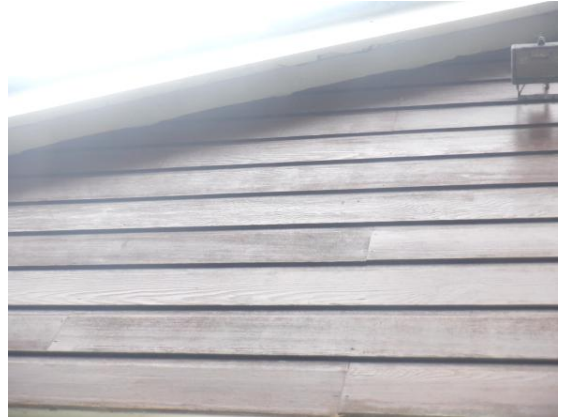
Photograph 13. Timber panels sealed along the edges of the gable (rear elevation).
