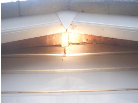
Photograph 14. Heavily cobwebbed gap at apex of porch (front elevation).
