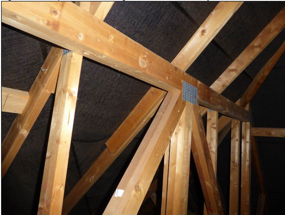
Figure 11. Example of bitumen lining. 21 Hubbard Close, Twyford, 30.07.24
