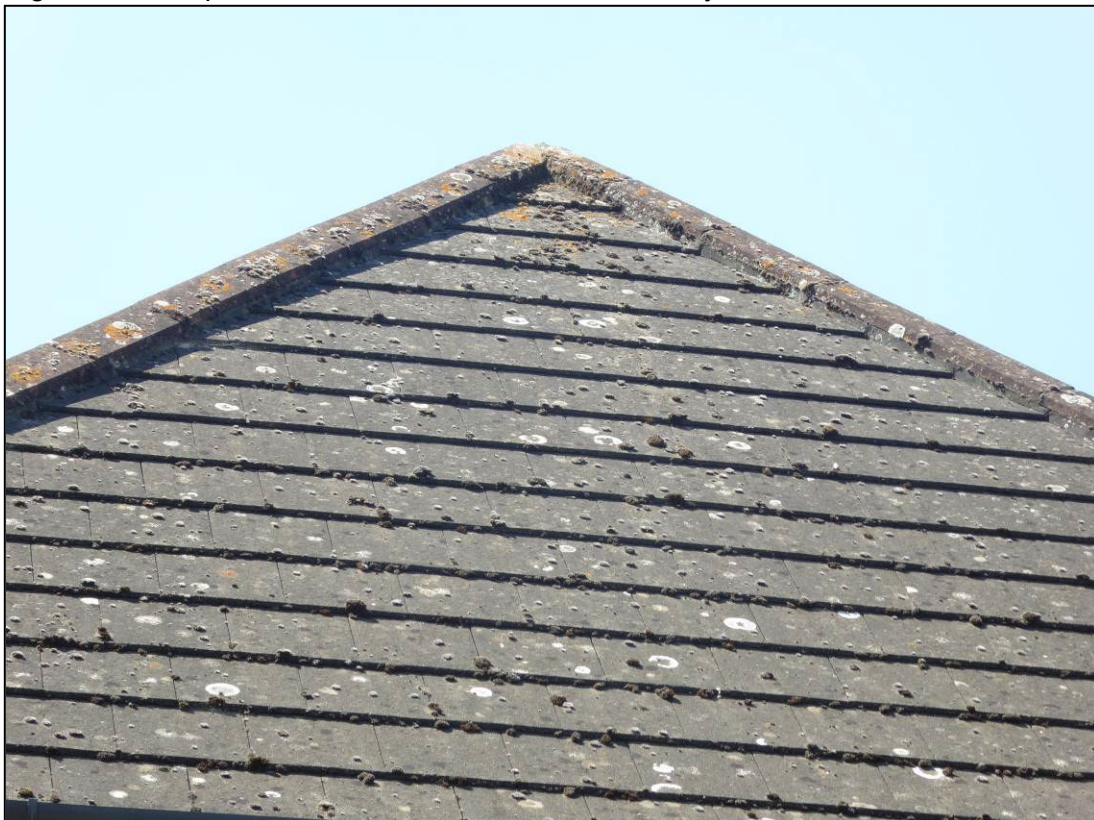
Figure 4. Example of roof tiles. 21 Hubbard Close, Twyford, 30.07.24
