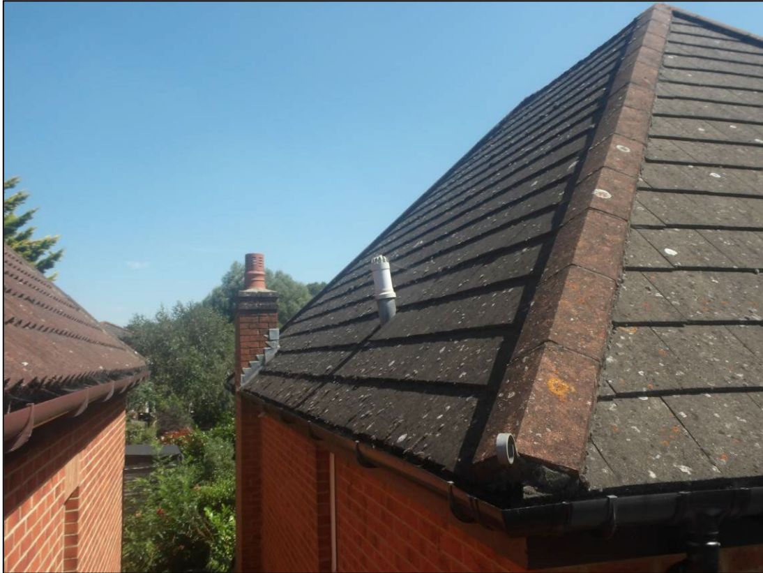
Figure 5. Example of hip tiles. 21 Hubbard Close, Twyford, 30.07.24
