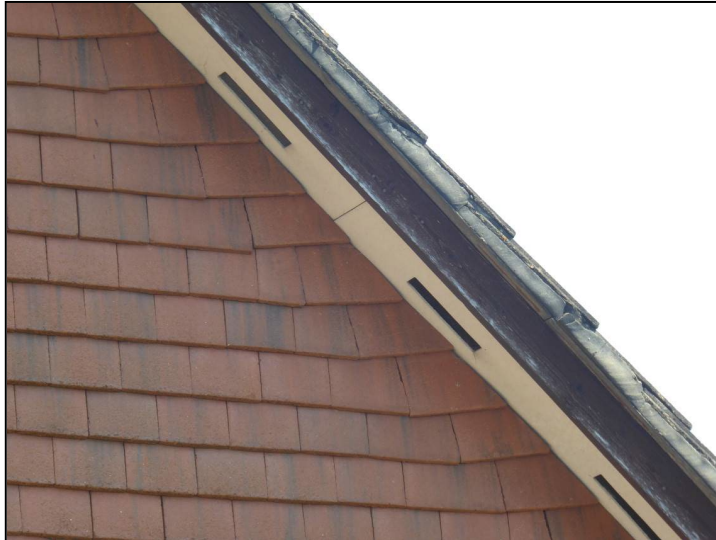
Figure 9. Example of hanging tiles. 21 Hubbard Close, Twyford, 30.07.24
