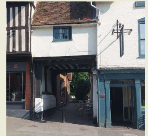
Figure 71: Typical covered passageway leading to courtyard
