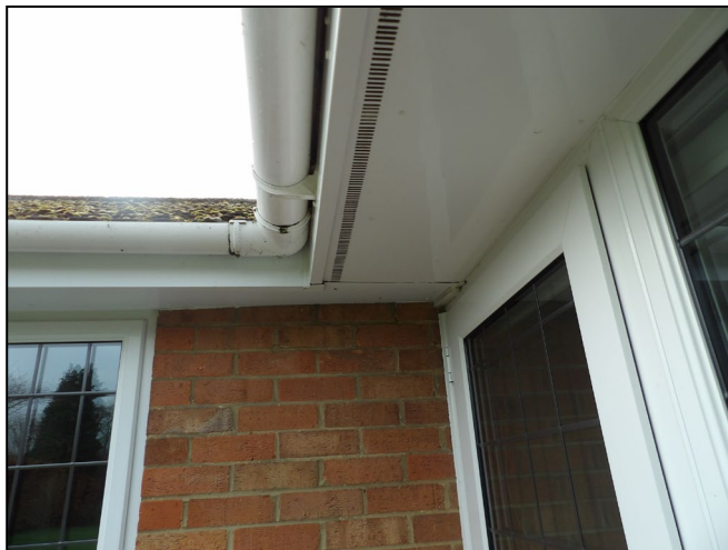
Figure 8. Example sealed uPVC soffits and fascias. 9 Northbury Avenue, Ruscombe. 21.01.25
