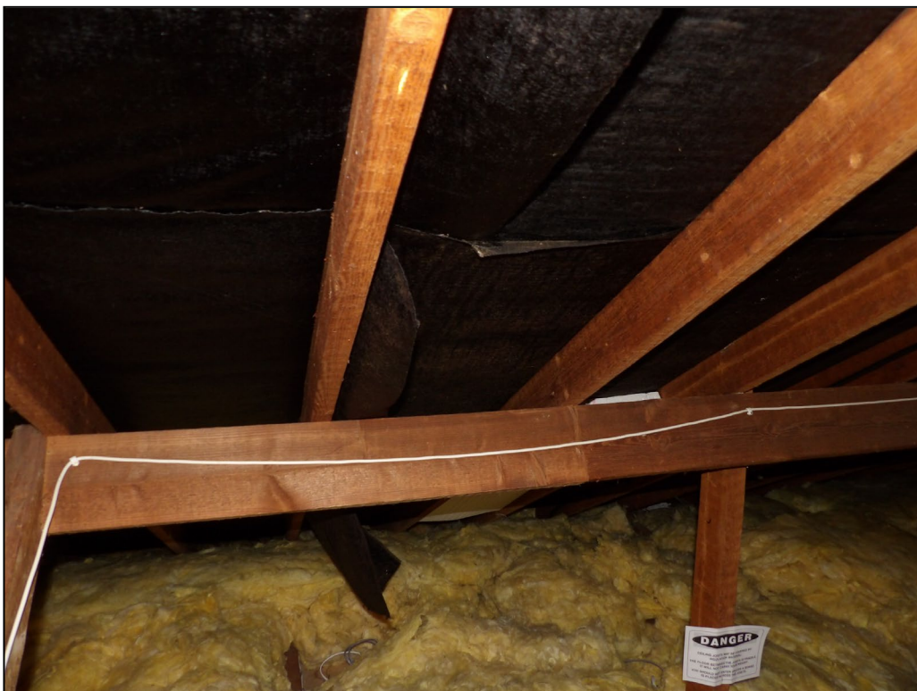
Figure 10. Example bitumen lining in main loft. 9 Northbury Avenue, Ruscombe. 21.01.25
