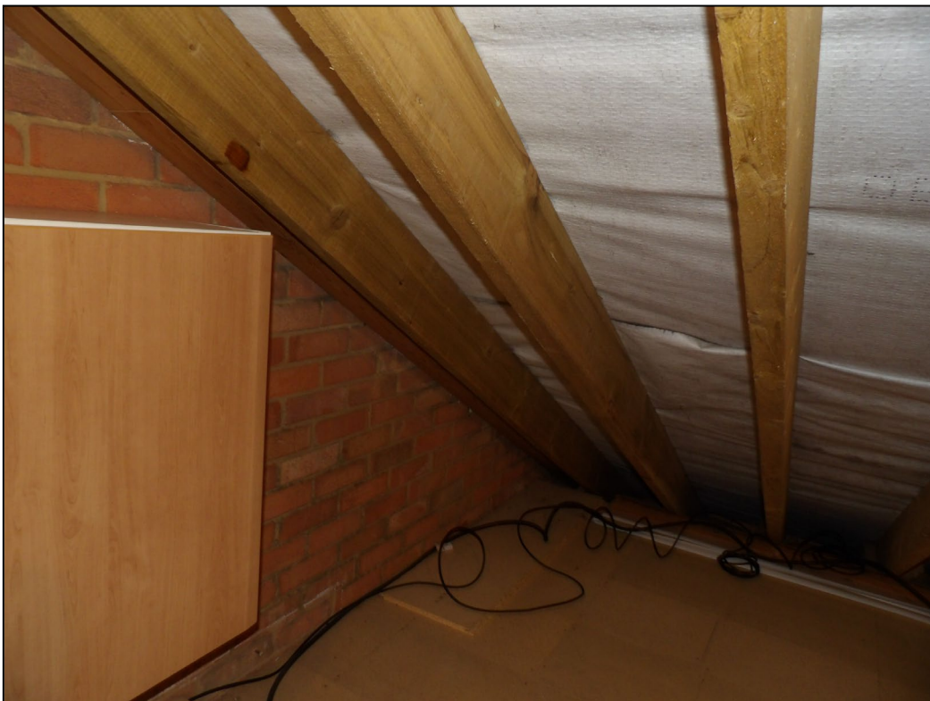
Figure 12. Membrane lining in second loft space. 9 Northbury Avenue, Ruscombe. 21.01.25
