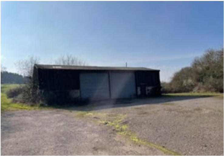
Existing building on site - to be removed.
