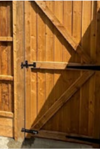
Timber framed, ledged & braced garden access gate
