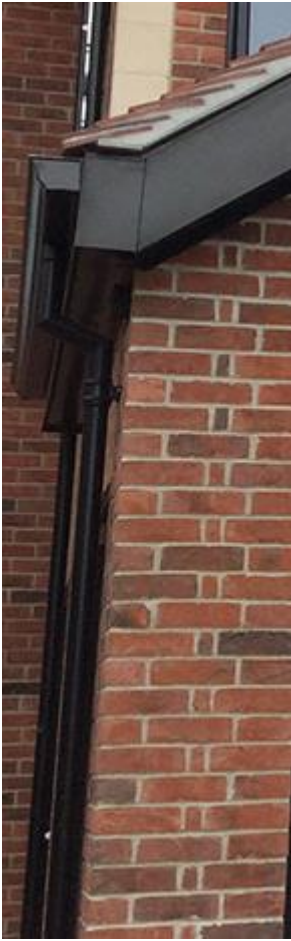
Black Painted Facia and guttering
