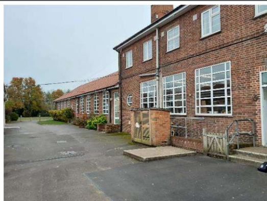
General site photograph.
