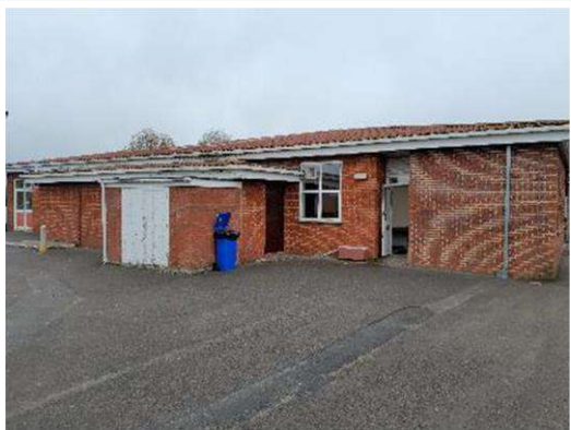
General site photograph.
