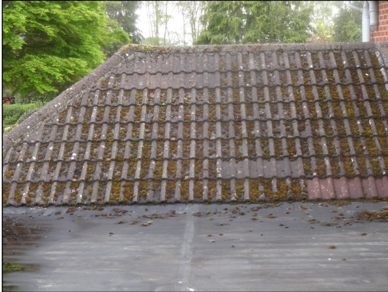
Figure 9. Roof, ridge and hip tiles of extension. 10 South Close, Wokingham. 15.04.25
