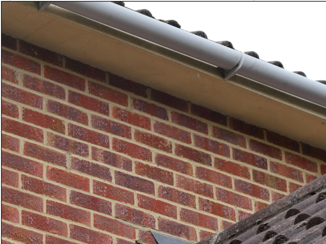
Figure 6. Example of soffits and fascias. 10 South Close, Wokingham. 15.04.25
