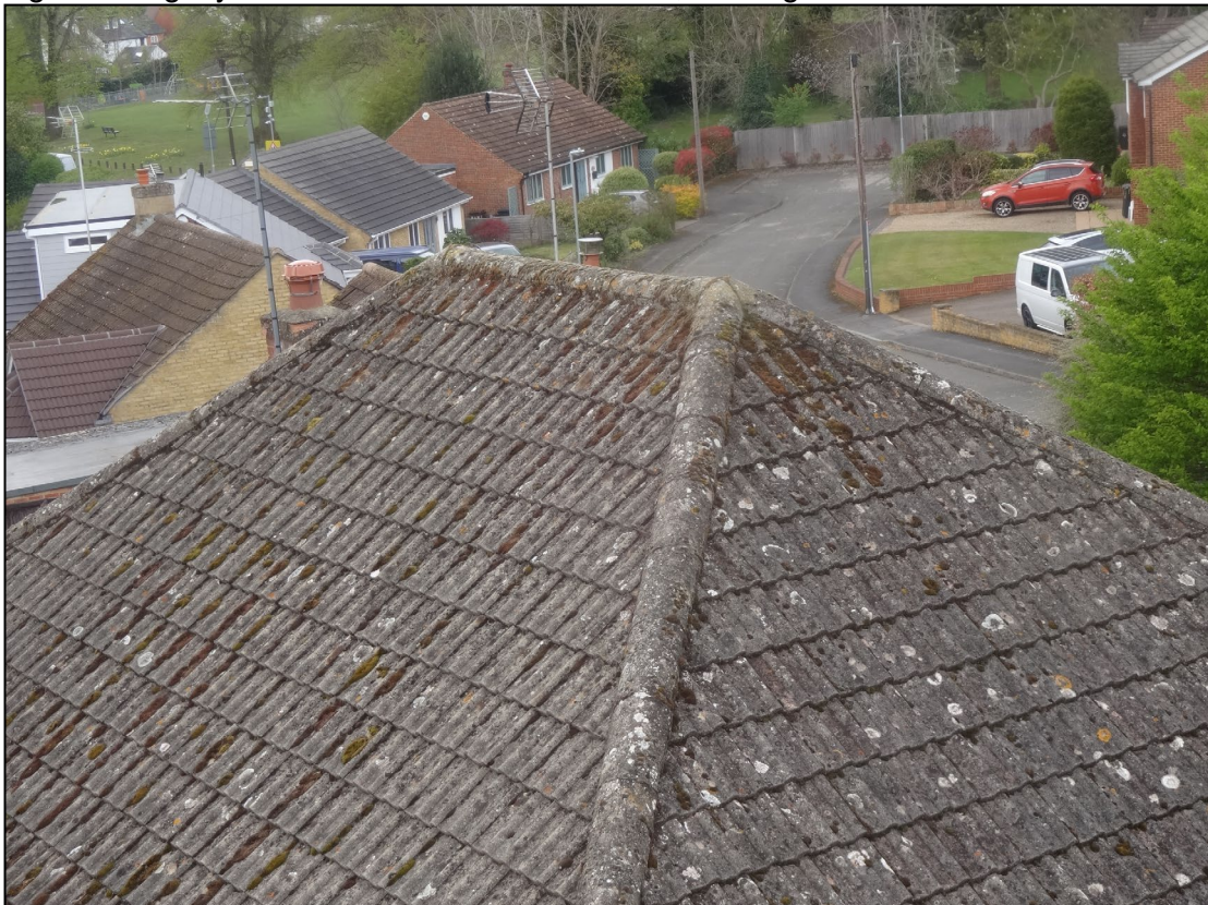
Figure 4. Tightly fitted roof tiles. 10 South Close, Wokingham. 15.04.25
