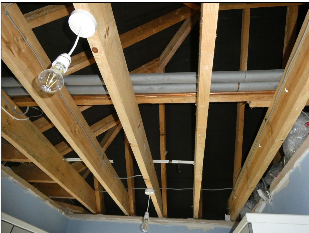
Figure 13. View of removed ceiling in hipped extension. 10 South Close, Wokingham. 15.04.25
