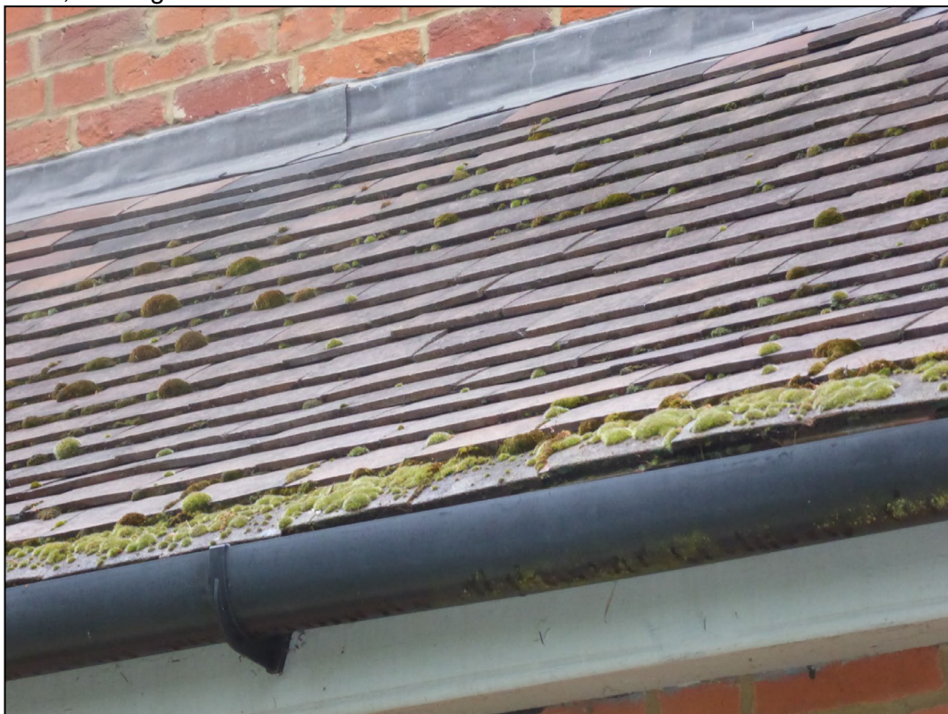
Figure 4. Example sealed tiles and lead flashing on single storey extension. 8 South Drive, Wokingham. 09.07.24
