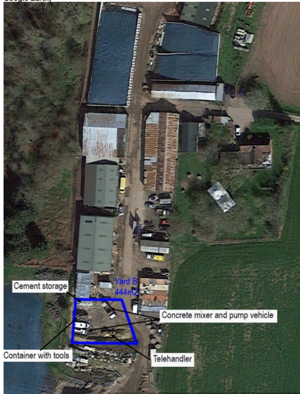
Aerial Photograph of Hill Farm dated 25 th March 2017 showing Yard B (Source – Google Earth)
