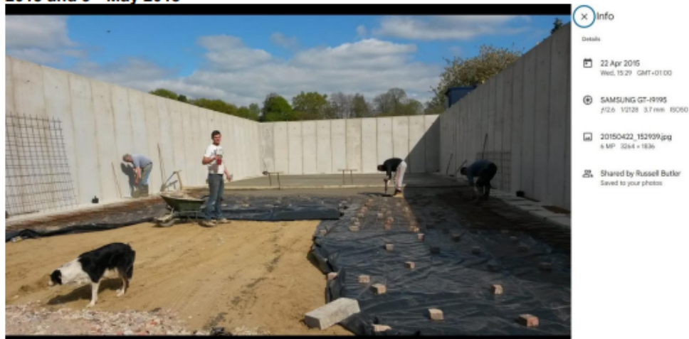
Photograph of Improvements to Silage Clamp (Previously Yard A) Dated 22 nd April 2015 and 9 th May 2015
