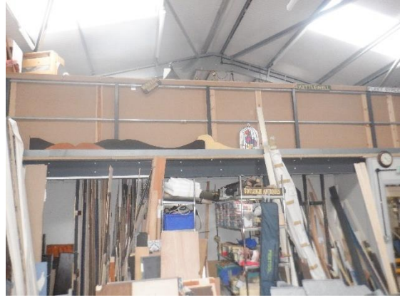
Photograph 33. Skylights within the roof of the store..
