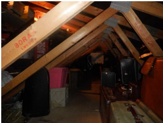
Photograph 22. Roof void 2 with trussed rafters.
