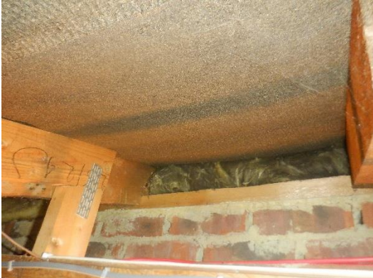
Photograph 26. Roof void 2 with fibreglass at the top of the walls.
