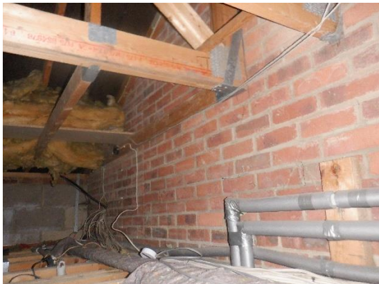
Photograph 27. Roof void 3 with trussed rafters with some raised sections covered with fibreglass, and lined with bitumen roofing felt.
