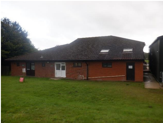
Photograph 13. Theatre viewed from south.
