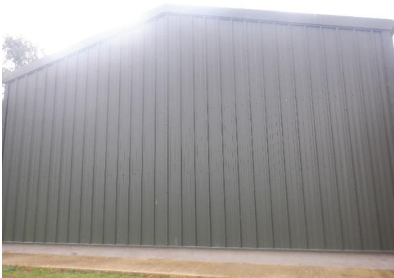
Photograph 31. Store of corrugated metal construction.
