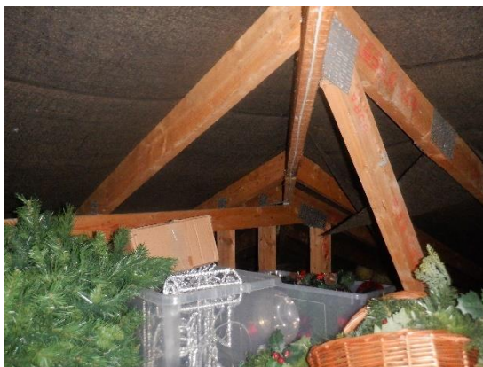
Photograph 24. Roof void 2 lined tightly with bitumen felt.
