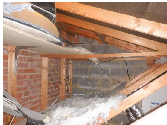
Photograph 25. Roof void 2 eastern gable end.
