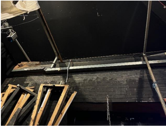
Photograph 30. The tightly fitted wall along the eastern side of the theatre.
