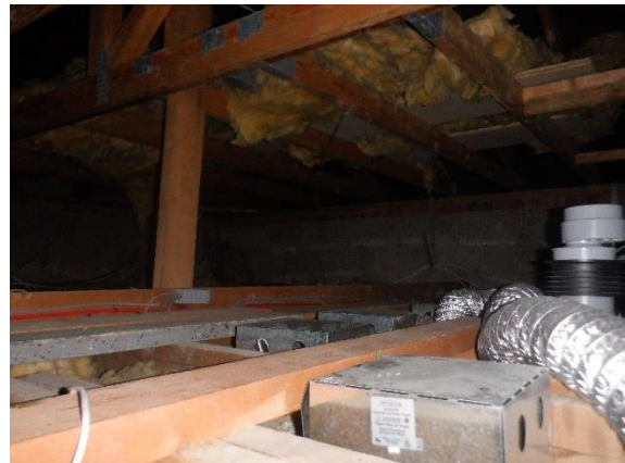
Photograph 28. Roof void 3 with an un-boarded floor.
