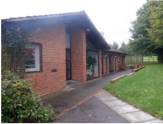
Photograph 8. Footpath around the theatre building.
