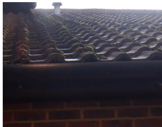
Photograph 16. Mesh along the base of the roof tiles.
