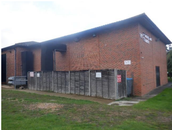
Photograph 7. Air conditioning units on the eastern side of the theatre.
