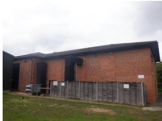
Photograph 14. Theatre viewed from east.
