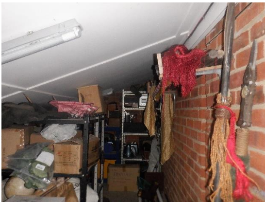
Photograph 19. Roof void 1 lined with timber.
