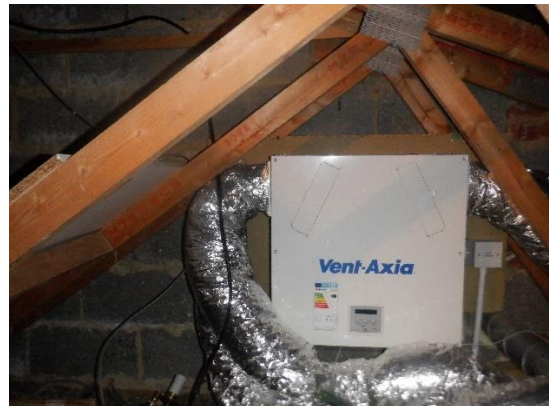
Photograph 23. Roof void 2 with a couple of vents.
