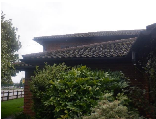
Photograph 15. Interlocking roof tiles and hip tiles tight (west elevation).
