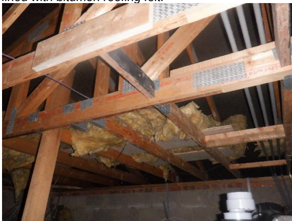
Photograph 29. Blockwork around the eaves in roof void 3.
