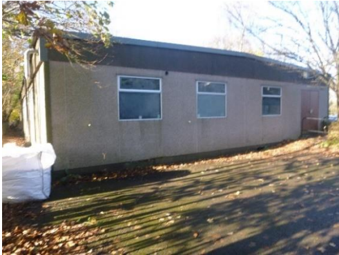
Photograph 1. Scout hut viewed from northeast.
