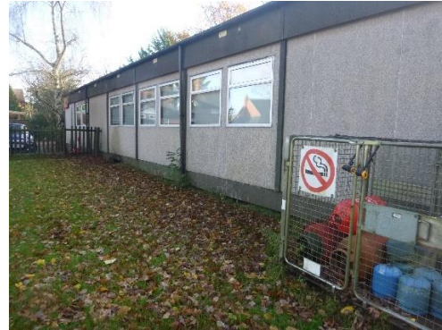
Photograph 2. Scout hut viewed from north.
