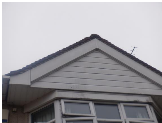
Photograph 7. Front gable fully sealed (front elevation).
