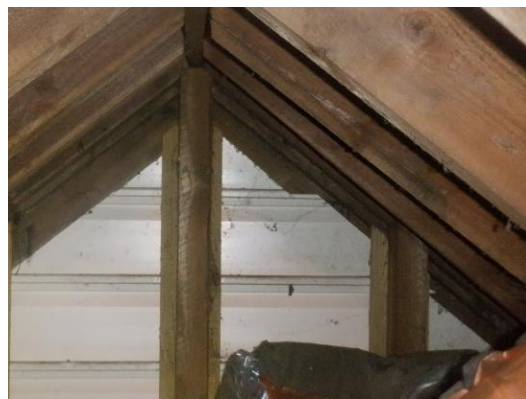
Photograph 14. uPVC cladding sealed to internal timbers.
