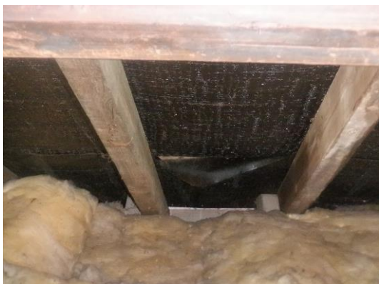
Photograph 13. Open eaves with access to uPVC soffit.
