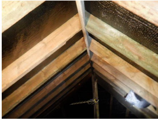
Photograph 10. Roof void of hipped construction with a cobweb free ridge.
