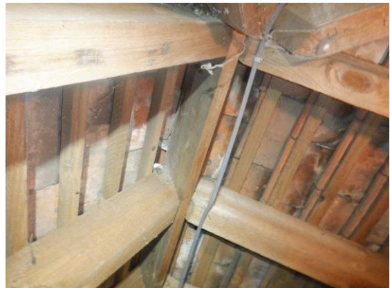
Photograph 12. Unlined roof at the eastern end (roof void).
