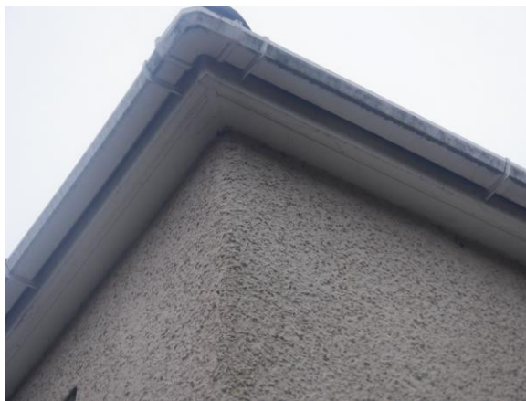
Photograph 8. uPVC soffit sealed to the rendered wall (rear elevation).
