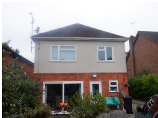
Photograph 2. Rear of property viewed from west.
