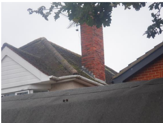
Photograph 6. Lead flashing sealed at base of chimney (north elevation).
