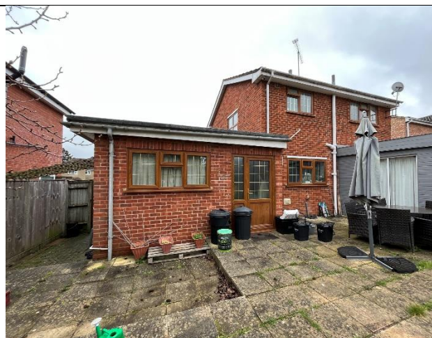
Photograph 2: The rear elevation.
