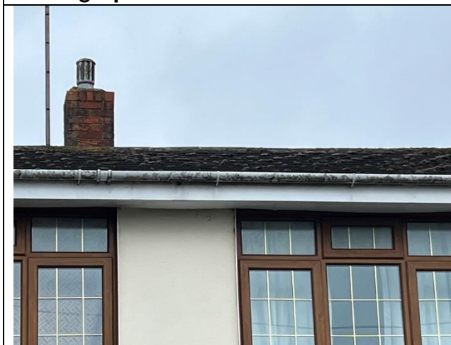
Photograph 3: Tight fitting roof tiles and soffits.
