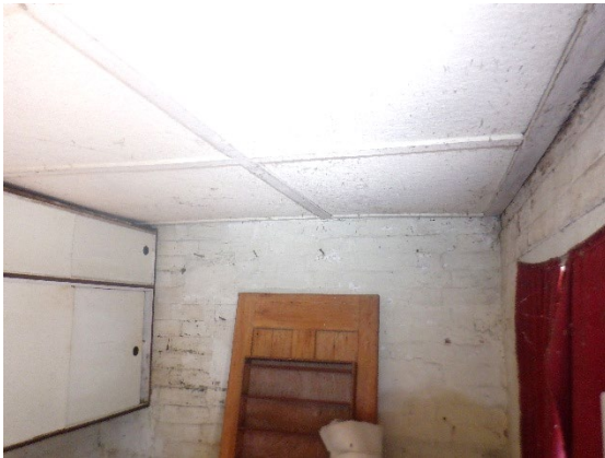
Photograph 11. The interior of the bathhouse showing hardboard ceiling and painted brick walls.
