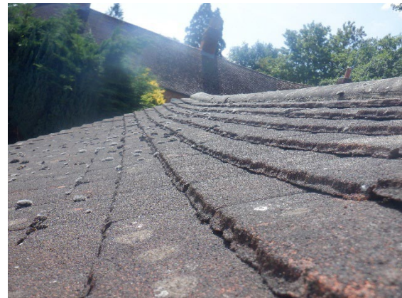
Photograph 4. Tightly fitted concrete roof and ridge tiles on most of the roof.
