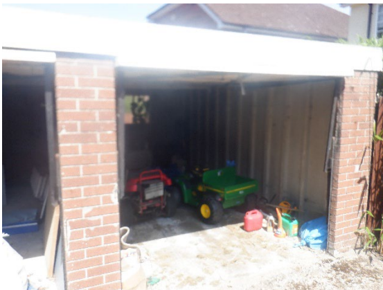
Photograph 7. Garage viewed from the front (east) showing up-and-over doors and dividing pillars.
