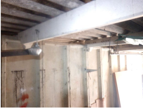
Photograph 13. The garage's prefabricated concrete walls, frame and corrugated sheet roof.
