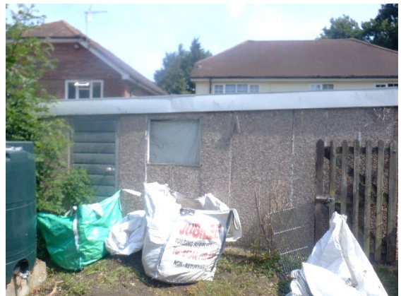
Photograph 8. The garage viewed from the side (south) showing the prefabricated concrete panels and uPVC fascias.
