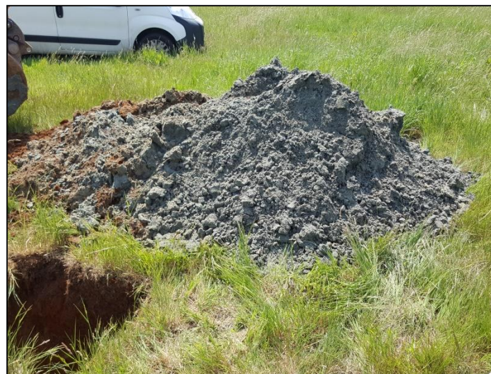
SA-02 excavated material
