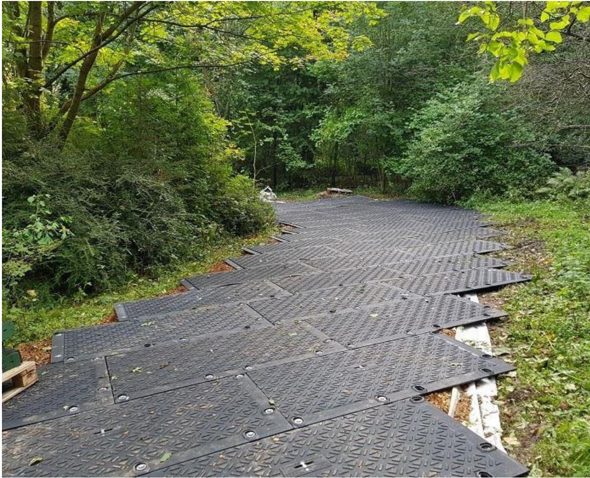
Figure 3: Example of ground protection to be utilised in the event the piling machine must access RPAs.
