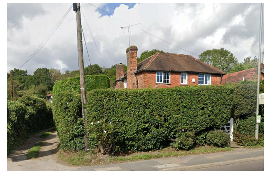
BOUNDARY TREATMENT AT PROPERTIES TO EAST OF PETROL STATION ON A4
