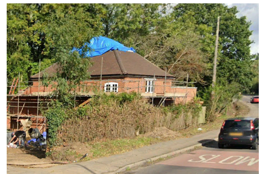
PRE- EXISTING FENCE WATERLOO COTTAGE (DURING CONSTRUCTION)
