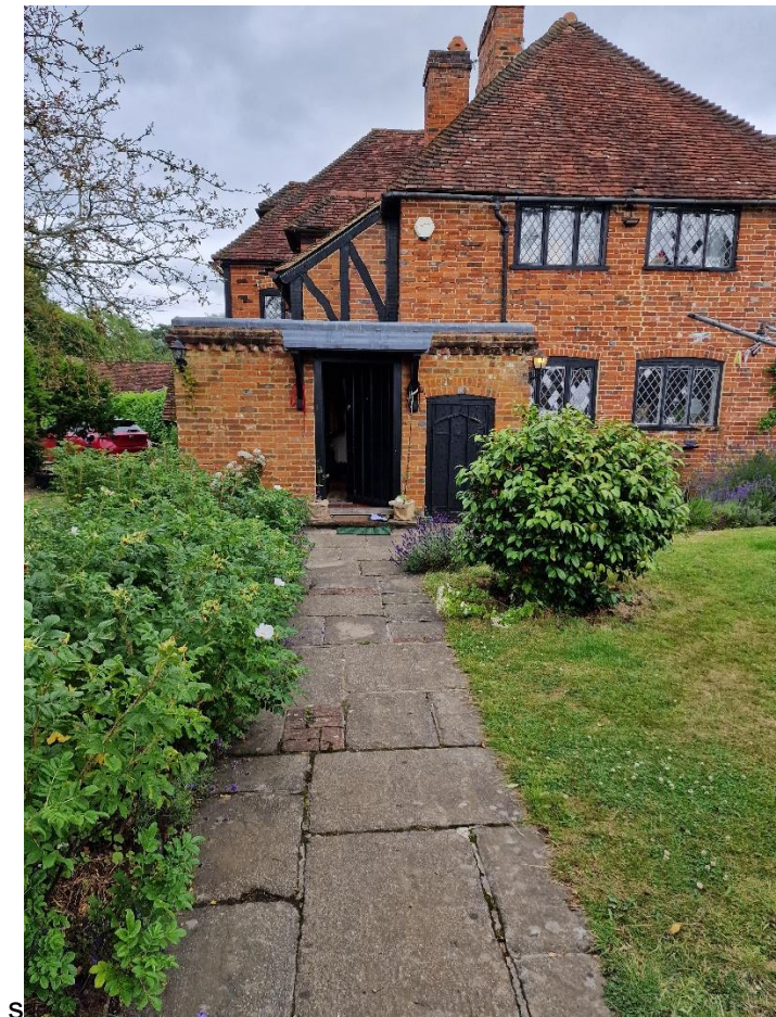
Existing Utility Room
