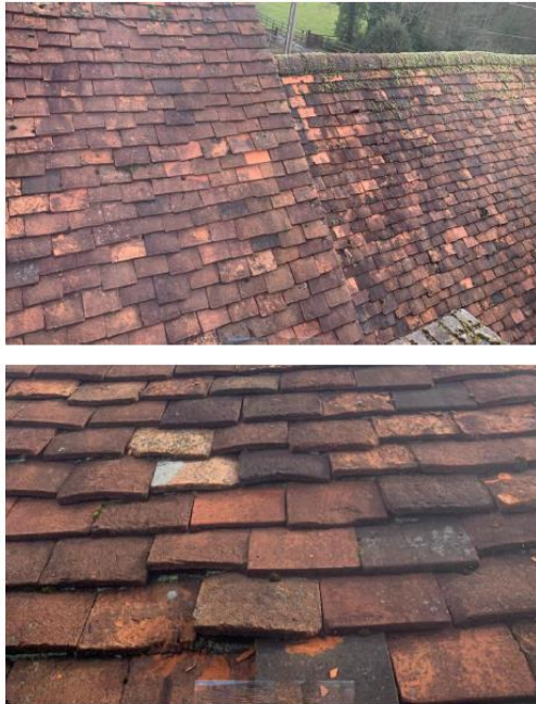
Additional images to show roof coverings to roost two and surrounding areas
