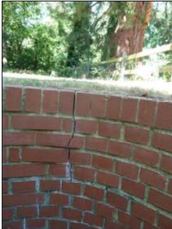
Photograph 2: Vertical crack, north west side, South Lodge, 30.6.2015.
