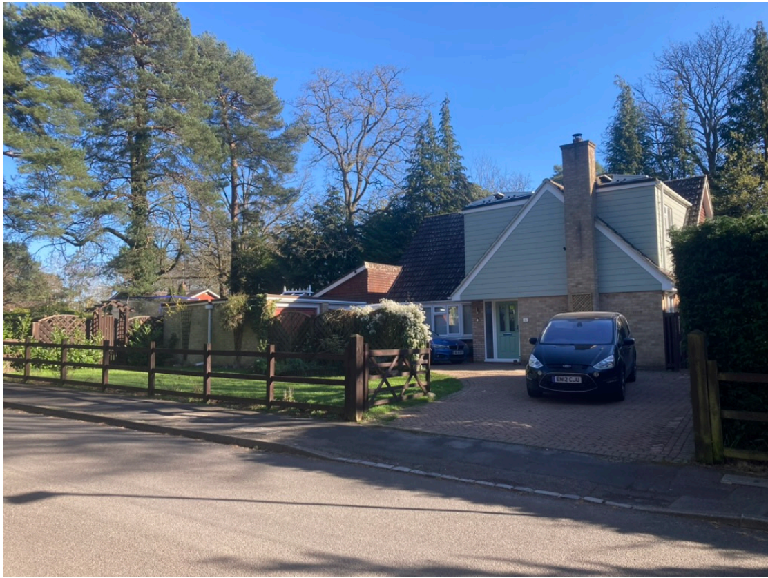
Figure 3 - 40 Linkway Front – Showing Existing Poor Roofline Above Dining Room
