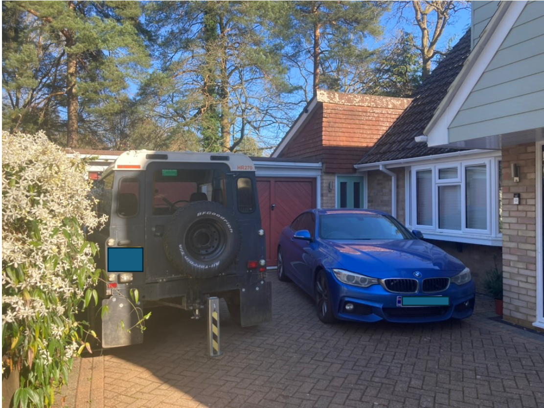
Figure 1 - 40 Linkway Garages & Existing Poor Roofline Above Dining Room
