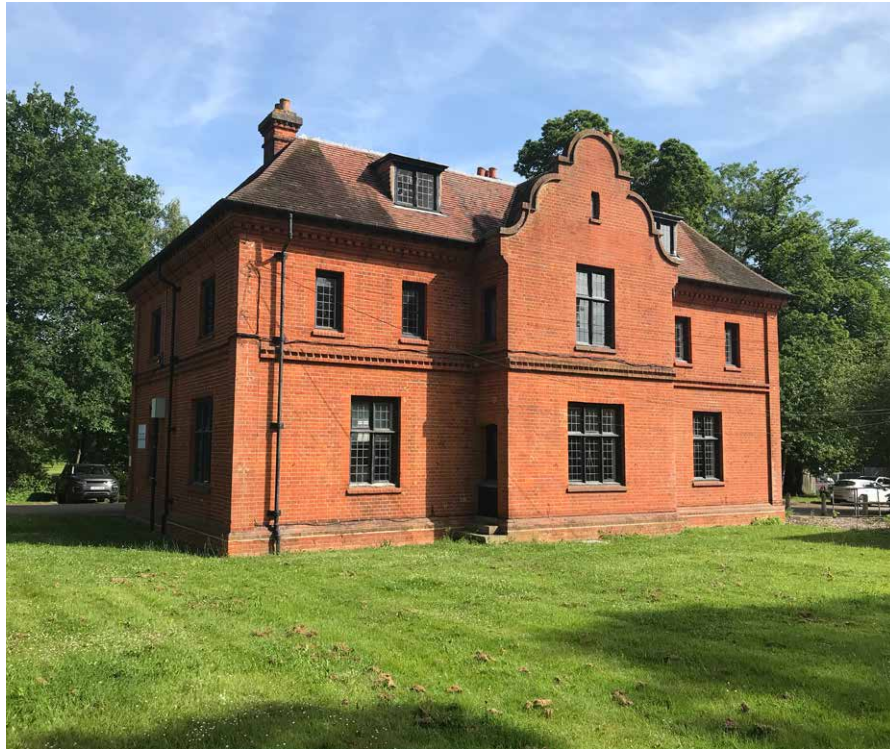
Figure 4.2 Moat House South Elevation
