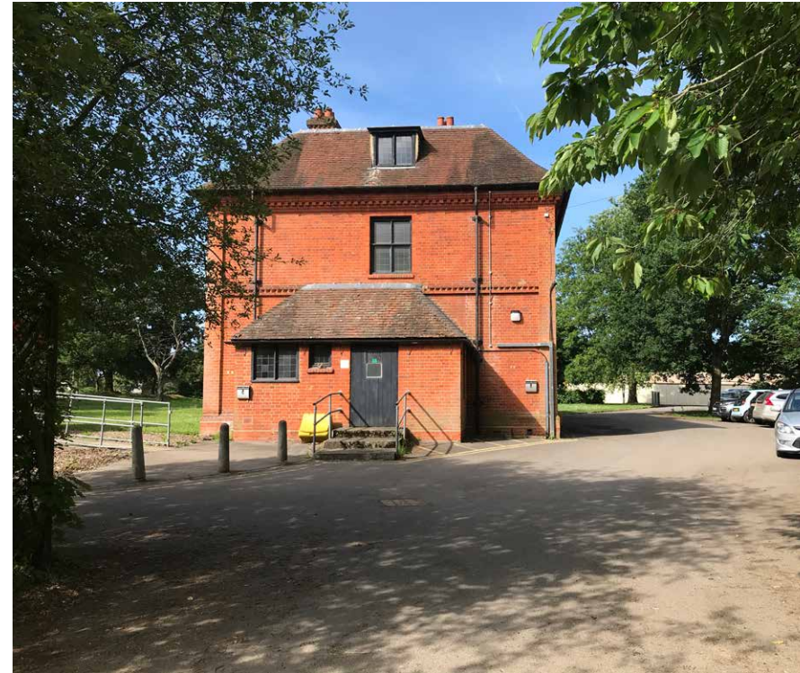
Figure 4.3 Moat House East Elevation
