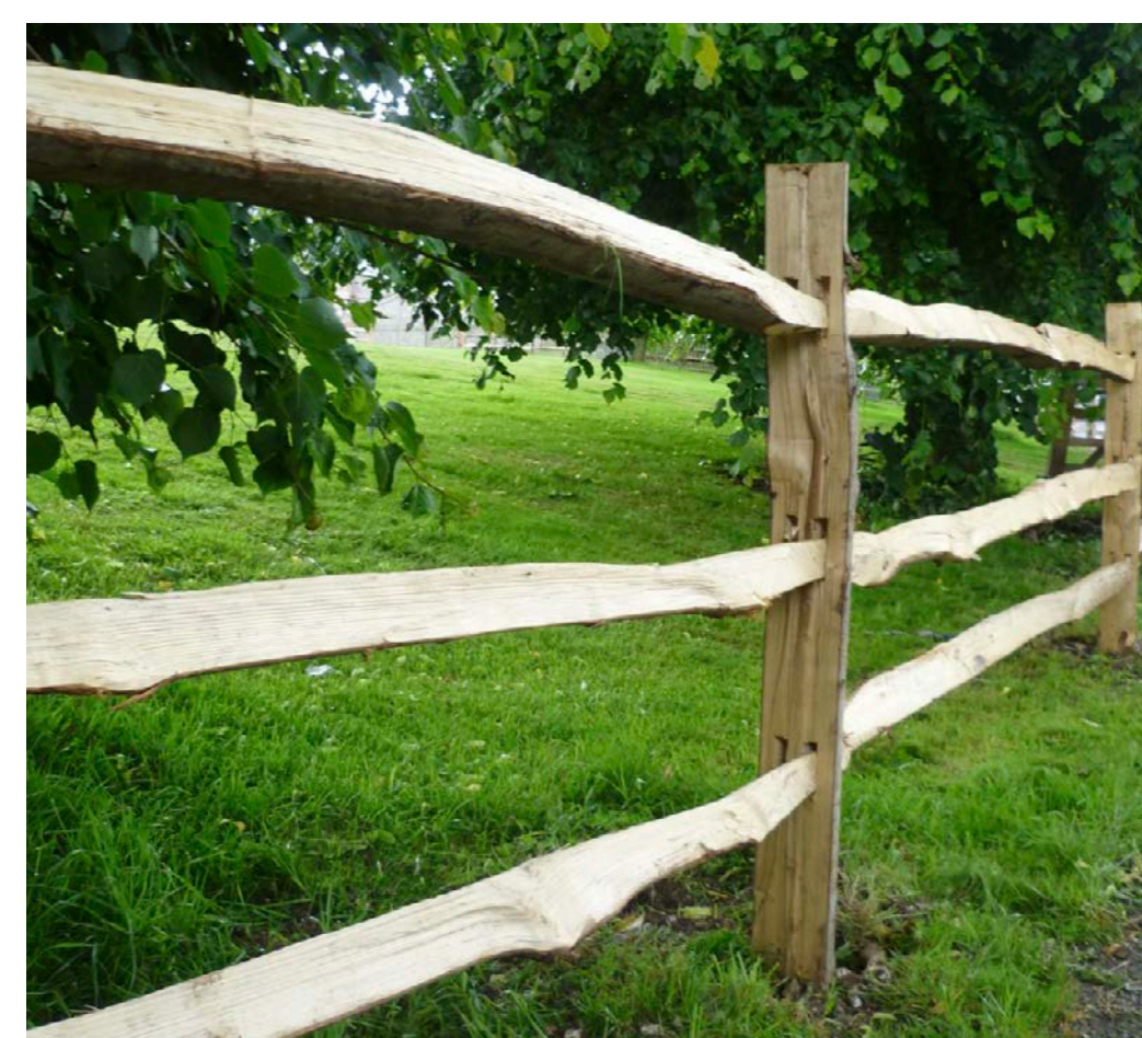
Cleft chestnut post and rail fencing
